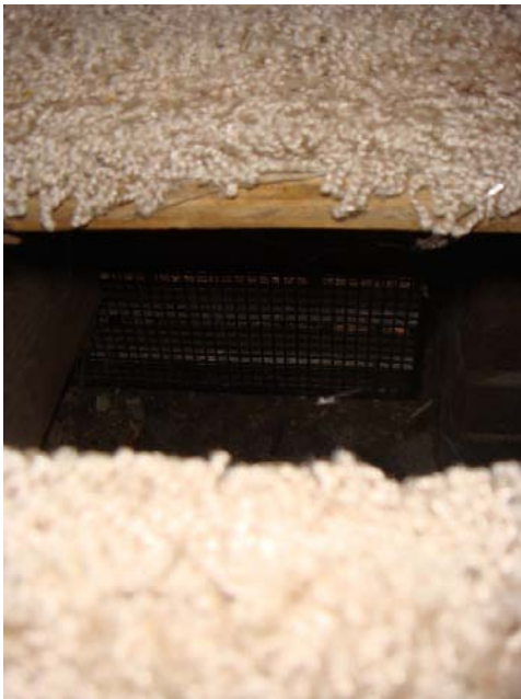
Figure 3. Crawl space viewable through living room register at disconnected duct
