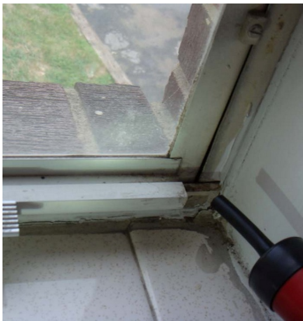
Figure 20. Window leakage
