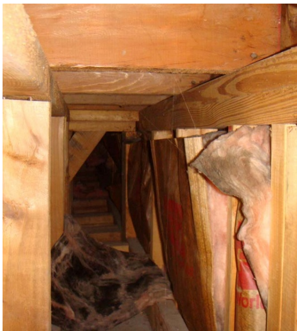
Figure 7. Inside kitchen soffit
