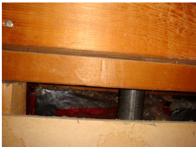
Figure 25. Plumbing penetrations into attic
