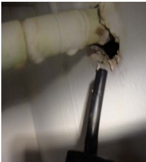
Figure 24. Plumbing penetrations
