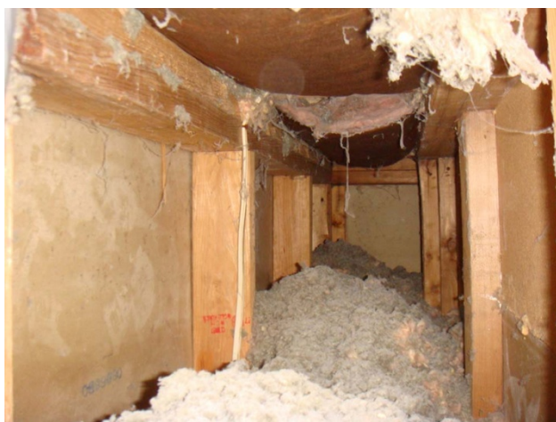
Figure 15. Open cavity between kitchen and living room
