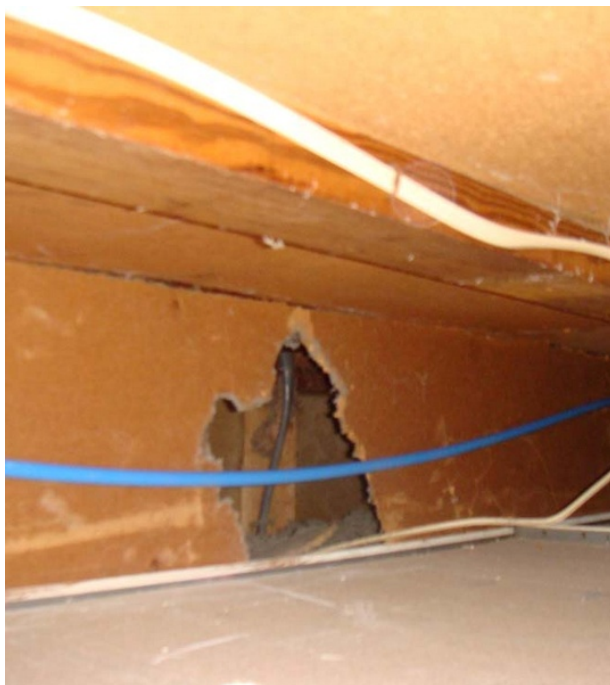
Figure 13. Semi-sealed dropped ceiling opening
