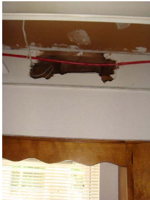
Figure 6. Dropped ceiling bypass into soffit over sink
