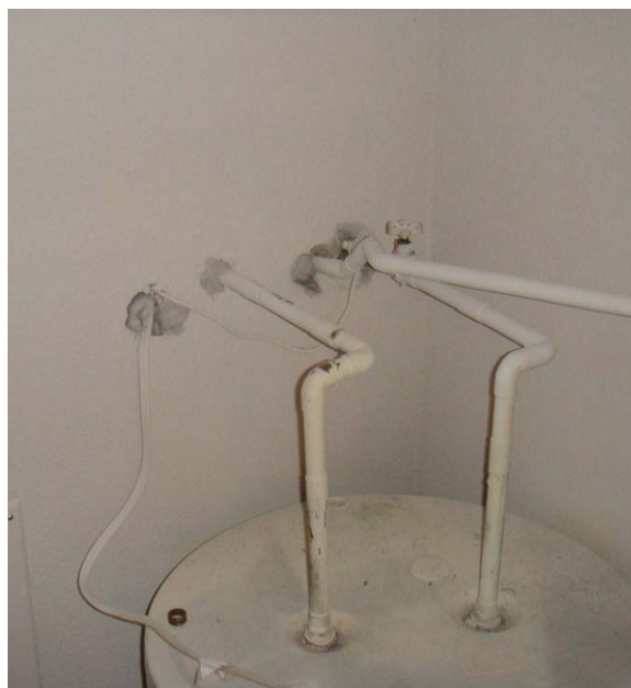
Figure 18. Water heater penetrations and hatch into plumbing access in bathroom closet
