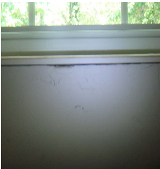
Figure 9. Gap under new window
