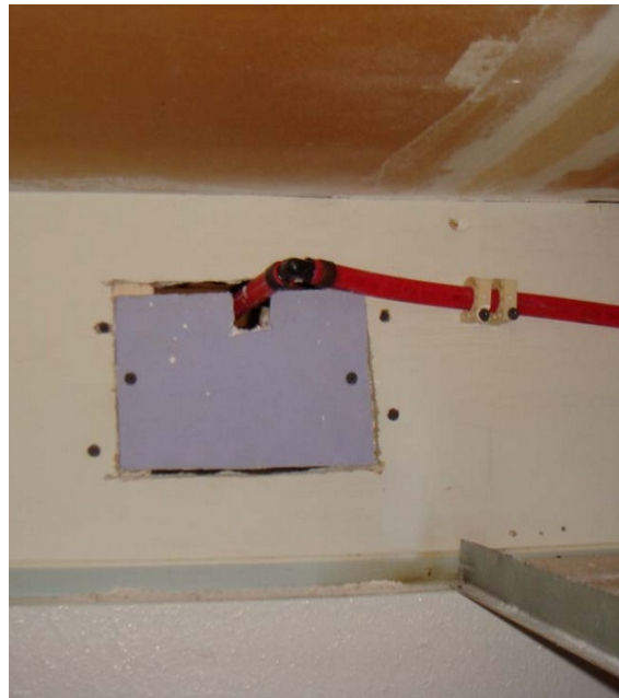
Figure 4. Dropped ceiling pipe penetration
