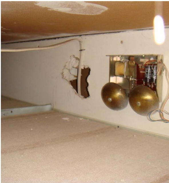
Figure 5. Dropped ceiling wire penetration
