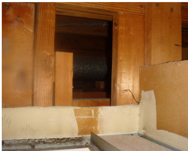
Figure 23. Open chase through dropped ceiling
