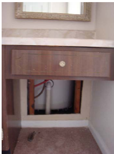
Figure 16. Hatch (opened to get picture) between bathrooms and plumbing penetrations
