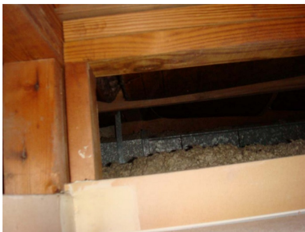
Figure 22. Open cavities through dropped ceiling
