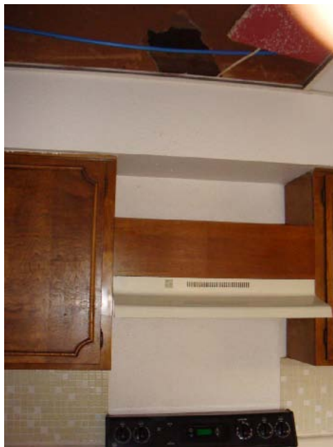
Figure 14. Semi-sealed dropped ceiling
