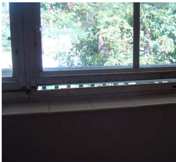
Figure 10. Window doesn't close
