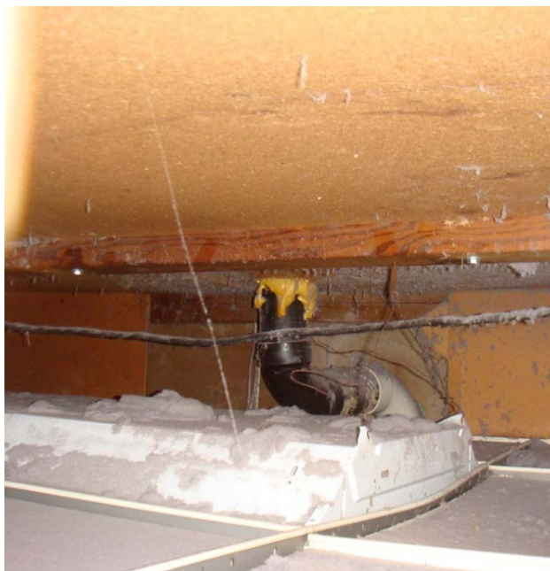
Figure 12. Semi-sealed dropped ceiling with pipe
