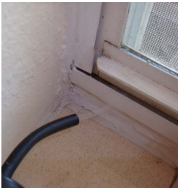
Figure 11. Window leakage
