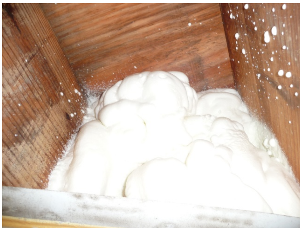
Figure 32. Floor joist cavity is sealed from vented eave.
