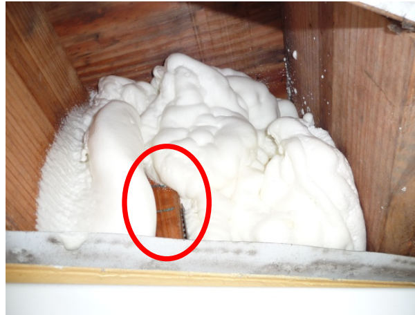
Figure 33. Spray foam expands considerably and conforms effectively around the end of a floor truss section within a floor joist.
