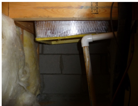
Figure 56. View inside a return plenum located in a garage. Air leaks are drawn primarily from the garage, but a small portion comes from the attic down through the wall cavity where the insulation is located. The block wall in the background is an exterior wall.
