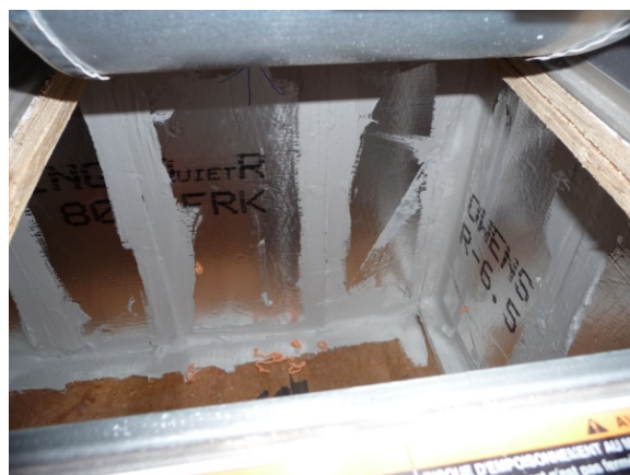
Figure 56. View inside a return plenum located in a garage. Air leaks are drawn primarily from the garage, but a small portion comes from the attic down through the wall cavity where the insulation is located. The block wall in the background is an exterior wall.
