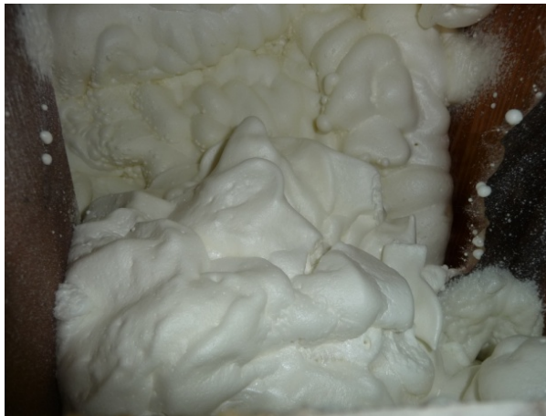
Figure 39. The next step is to complete the seal from floor deck vertically down to the bottom of the soffit surface. This is done between each joist section.
