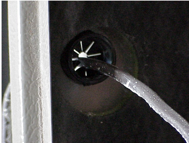
Figure 48. Leaky thermostat wire penetration.
