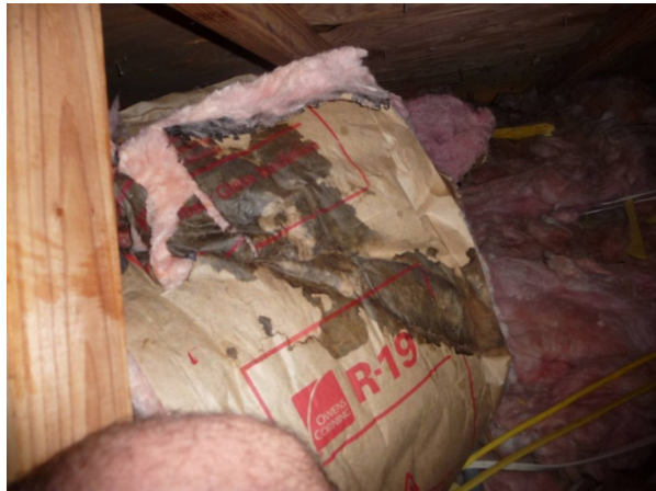
Figure 41. Batt pulled away from duct shows it is soaked where dark areas are seen on paper facing.
