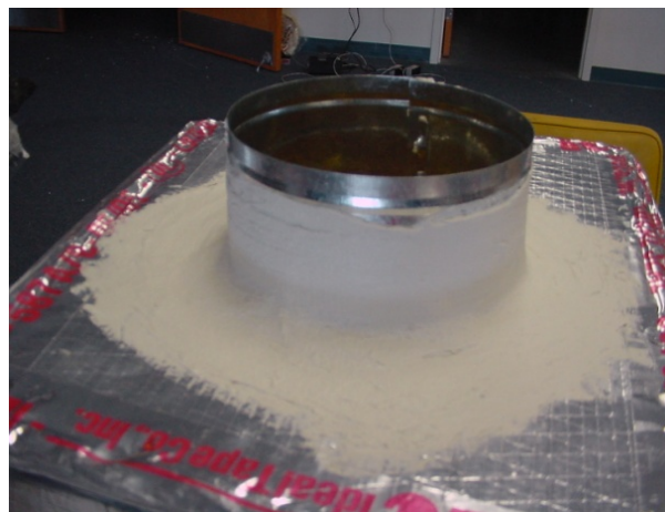
Figure 64. Apply mastic from the foil surface of duct board over and around the metal collar. Mastic can be applied over any securely bound tape.
