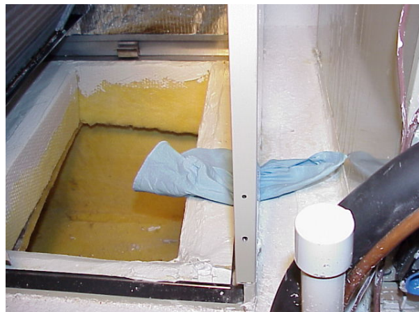
Figure 51. Blue cloth has been pulled under AHU cabinet to illustrate air pathway where the return plenum and the AHU join together.
