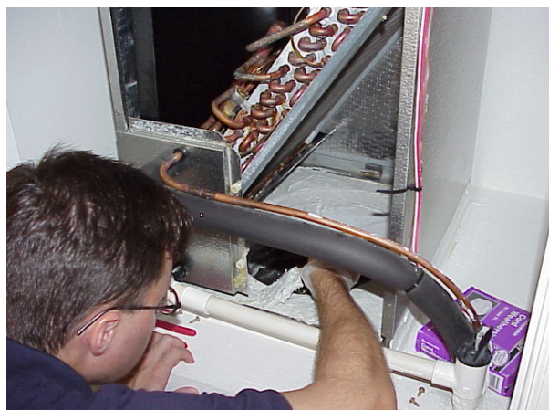
Figure 52. Duct mastic applied in a continuous seal from return duct air barrier to the AHU air barrier. Use care not to get mastic on the coil or any removable panel seam.
