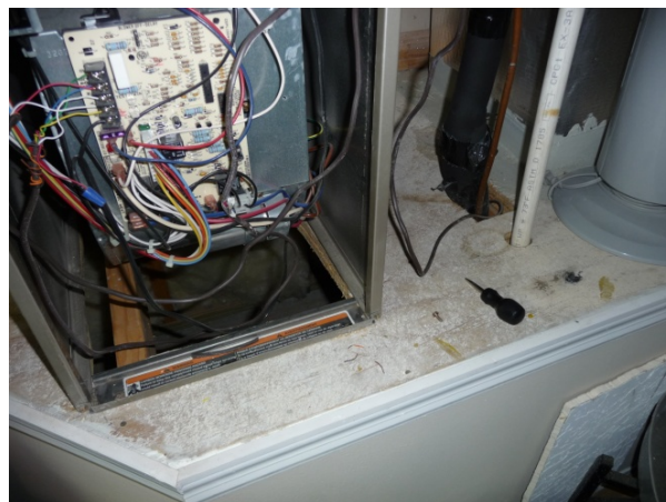
Figure 54. Front panel of furnace is removed for inspection inside the return plenum. Because of limited plenum access, part of the drywall has to be removed to provide access for plenum sealing.
