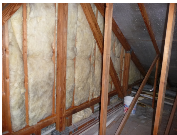
Figure 21. View of kneewall and portions of open floor cavity as seen from inside the garage attic.
