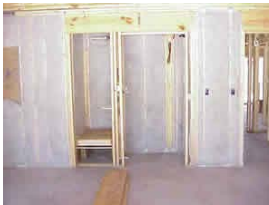
Figure 16. An insulated garage closet located will house an AHU. A weather stripped door will isolate the closet from the garage. A vent from the closet to indoors would also further enhance the system operating efficiency.
