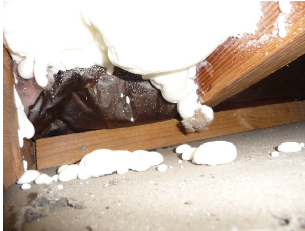
Figure 38. First, the foam spray gun is inserted into the soffit vent hole to apply foam insulation to the floor deck above, beyond the top of the exterior wall.
