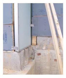
Figure 19.1. Seal air gaps between two framed common walls (Source: Energy Services Group, from EPA 2008)
