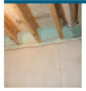
Figure 17.2. Spray foam along the basement rim joist to provide a complete air barrier connecting the foundation wall, sill plate, rim joist, and subfloor (Source: BSC 2009C).
