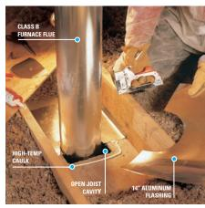
metal dam should be used to keep insulation away from the flue. The same technique is used for masonry chimneys.
