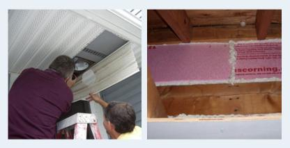
Figure 7.1. When researchers pulled back the porch ceiling, they found the wall board was missing so nothing was covering the insulation on this exterior wall. An air barrier of rigid foam board was put in place with spray foam (Source: Moriarta 2008).
