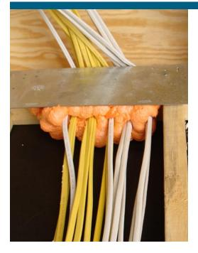
The holes in the sill plate were properly air sealed during construction of this house.
