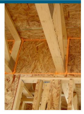
15.2. Seal rim joists of the wall separating the house's living space from the garage with pieces of wall board and spray foam.
