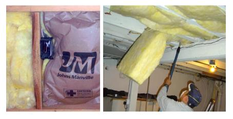
Figure 1.1. *(left)* Cut fiberglass batt insulation to fit around electrical boxes and wiring or pipes that run through the walls. Compressions like these ruin the batt's thermal alignment with walls and lessen its effectiveness.
