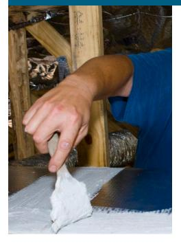
Figure 11.1. Paint mastic (a thick, gooey substance) on to the duct seams and joints. (Photo source: Habitat for Humanity Lakeland FL).
