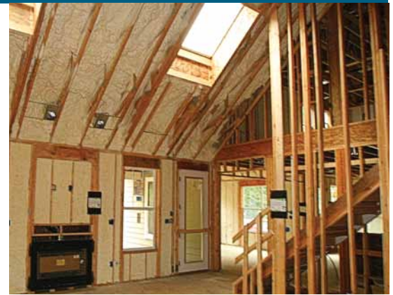
The walls, ceilings, and rim joists are insulated with spray foam, which provides insulating and air sealing properties.
