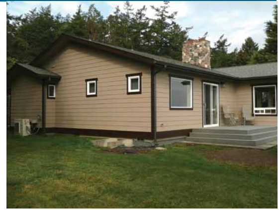
Visible here on the home's southeast side is one of the outside units for the ductless heat pump system that replaced the home's ancient furnace and leaky ducts, providing efficient, ductless, zoned heating and cooling.
