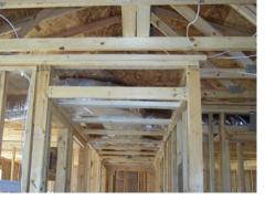
Keeping the airhandler and ducts in conditioned space such as this chase reduces outside air leakage and prevents temperature differences inside and outside the ducts, that can lead to condensation and mold problems.
