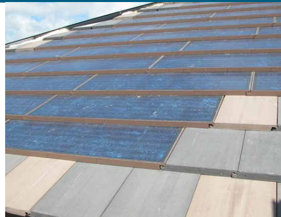
Solar photovoltaic roof panels mirror the size of cement roofing tiles for a nearly invisible appearance on LifeStyle's luxury zero-energy home.
