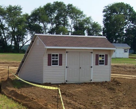
New Jersey builder Mark Bergman combined Building America building science know-how and a personal commitment to energy efficient construction to achieve energy savings of 46% over the Building America benchmark home. (Above) Wiring for the photovoltaic system runs underground from the sheds to the houses.
