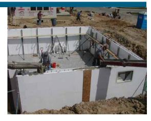
Insulation beneath the concrete slab and insulated concrete forms for the lower walls contribute to a tight thermal envelope for this home near the shores of Lake Michigan. Extensive air sealing creates a comfortable, energy-efficient haven in a climate with cold, windy winters and hot, humid summers.
