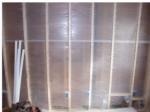
(top) The double-stud wall consists of two 2x4 16-inch-on-center framed walls set 5 inches apart.
