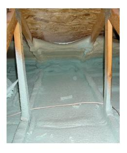
Spray foam is used to insulate and air seal the attic floor and any ducts located in the attic. The spray foam is covered with more than 12 inches of blown cellulose for the equivalent of R-49 of attic insulation.
