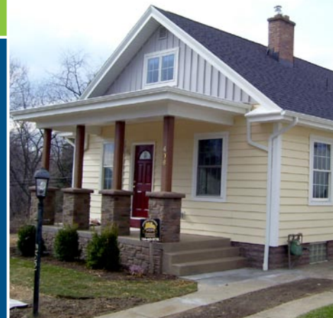
Asdal Builders achieved a HERS score of 65 and cut energy use by 80% with a gut-rehab of this 1930s era Pittsburgh home.
