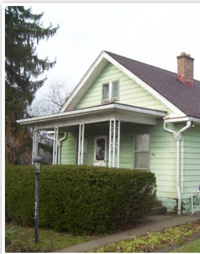
Pittsburgh home pre-retrofit.
