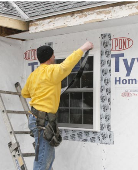
Energy-efficient windows were flashed and integrated into the housewrap.
