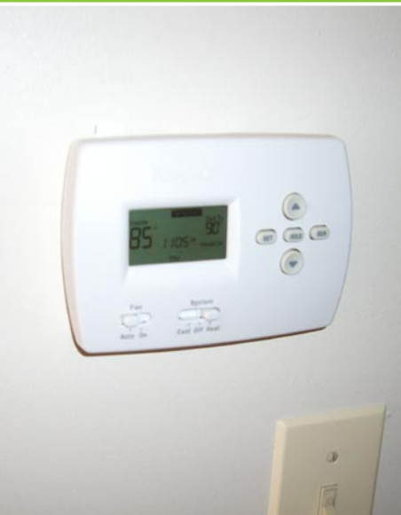
(left) Programmable thermostats.
