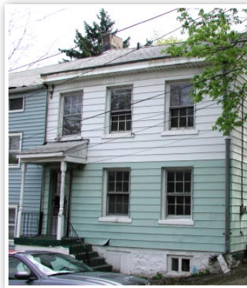
85 Nicoll St. pre-retrofit.
