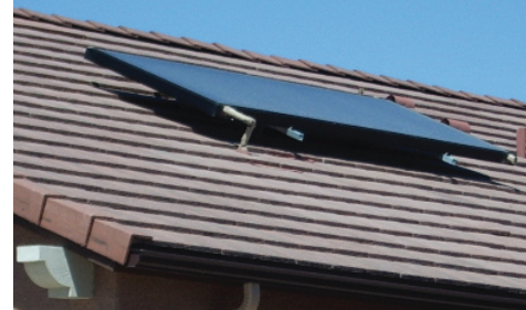
With help from Building America research, Pulte selected closed-loop, active solar water heating units.
