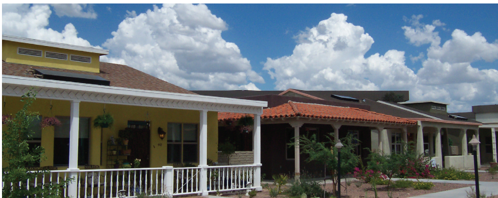
Copperheart Integrated Collector Storage water heaters are included on each JWM house. Photo courtesy of the Solar Store.
