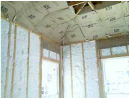
Continuous formaldehyde free fiberglass blown insulation
