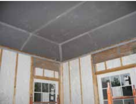
Sealed drywall at ceiling
