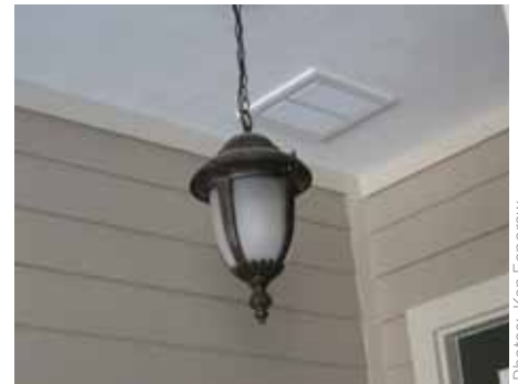
Outside air inlet with filter back grille delivers fresh air to return side of AHU
