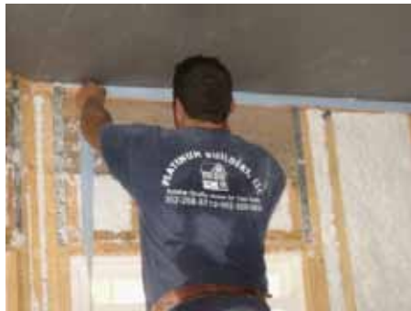
Foam gasket at ceiling/wall joints ensures airtightness
