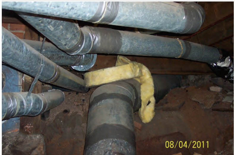
Uninsulated, partially sealed ductwork in the uninsulated basement/crawlspace
