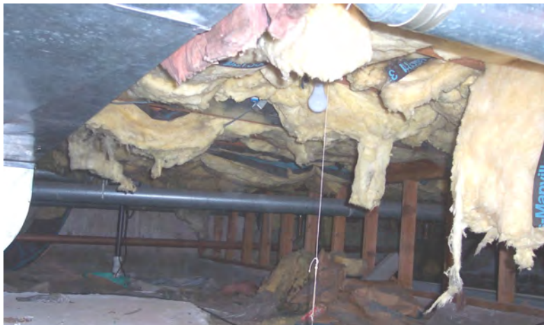
All ductwork and the heating system were located in the vented crawlspace. Insulation was falling down in multiple locations.
