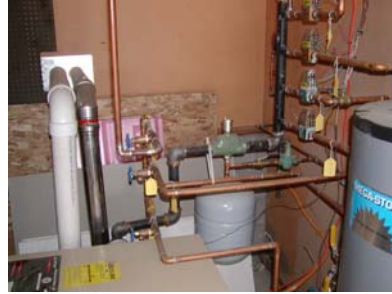
Sealed Combustion Boiler
