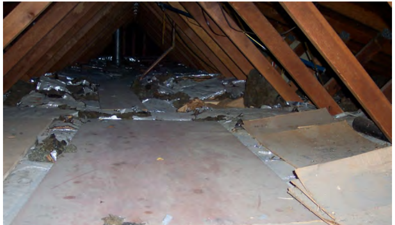
Attic is only insulated to R-11.
