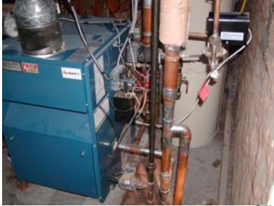
Atmospheric Gas Boiler
