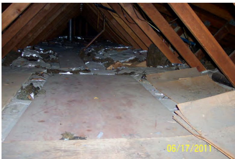
Attic is only insulated to R-11.
