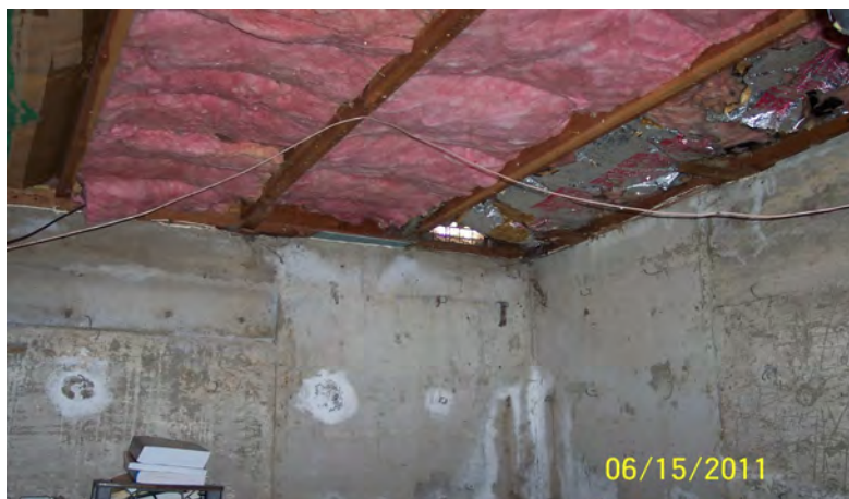
This home receives no credit for the crawlspace ceiling insulation because the majority of the ductwork is located here.
