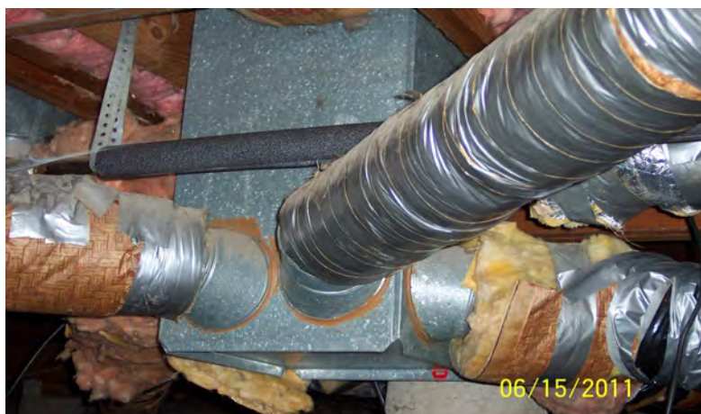
Main supply plenum from down flow furnace with supply branch takeoffs. 99% of the supplies are located in this crawl.
