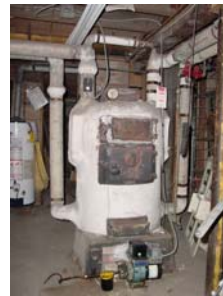
Coal-Conversion Boiler
