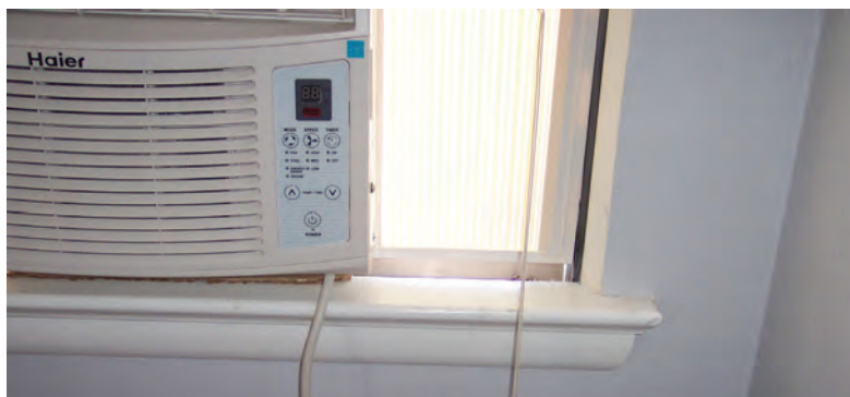
A window air-conditioner was installed after the initial SmartRegs inspection. A large air-gap around the A/C resulted in a significant increase in the overall infiltration rate of the apartment.
