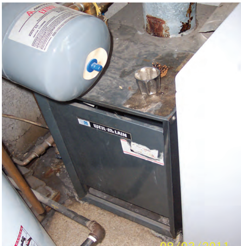
Replacing this 60% efficient gas boiler with a 90% efficient unit gains 17 points on the SmartRegs checklist. Installing 1 kW of PV is awarded 44 points.
