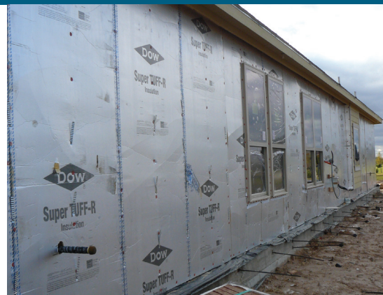
David Weekley Homes covers the building exterior with 1-inch of rigid foam XPS providing a continuous air barrier and thermal break for the building envelope.
