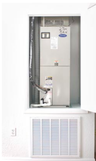
Figure 22.2. An alternative to a closet located in the garage is an in-house location. (Photo courtesy of FSEC)
