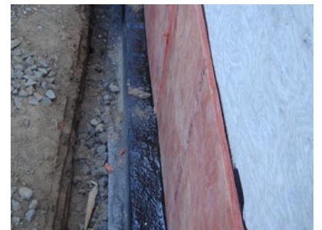
Figure 2.4. Example of damp proofing and exterior insulation below grade
