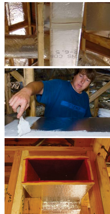
Figure 15.1. Mastic provides the most reliable duct sealing method. Ducts should be located in conditioned space.
