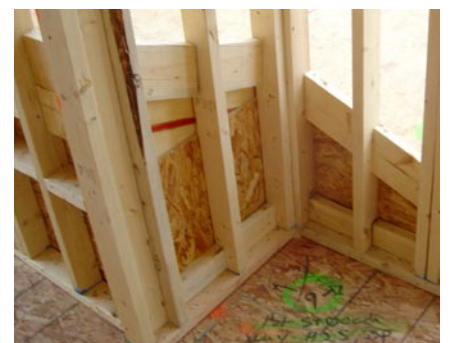
Figure 16.2. Sequence framing to install an air barrier between the porch roof cavity and conditioned space.
