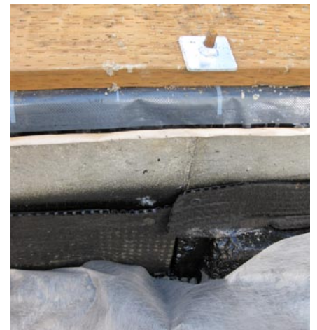
Figure 2.4. Example of damp proofing and exterior insulation below grade
