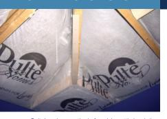
Pulte's unique method of applying attic insulation keeps the blown cellulose right up against the roof line providing an insulated attic providing conditioned space that hovers around 80°F to house the air handler and ducts instead of the 150°F temperatures found in uninsulated Las Vegas attics.
