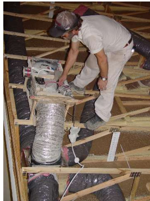
Duct testing rig at Palm Harbor Homes, Plant City factory, Florida
