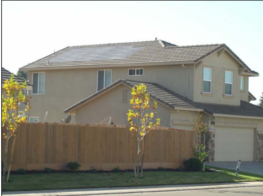
At ground level, BIPV blend in well with roof tiles.
