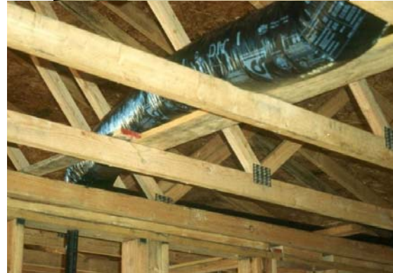
Ducts in a California home moved to the attic floor.
