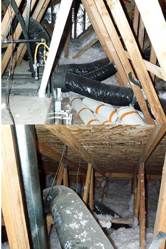
Ducts in the attic of a model home. Although buried ducts were specified, only one branch is buried to any degree. Most ducts are hung or otherwise above the insulation.
