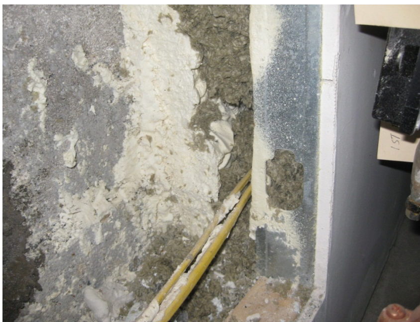
Figure 4. Belmont Two-Family basement wall insulation
