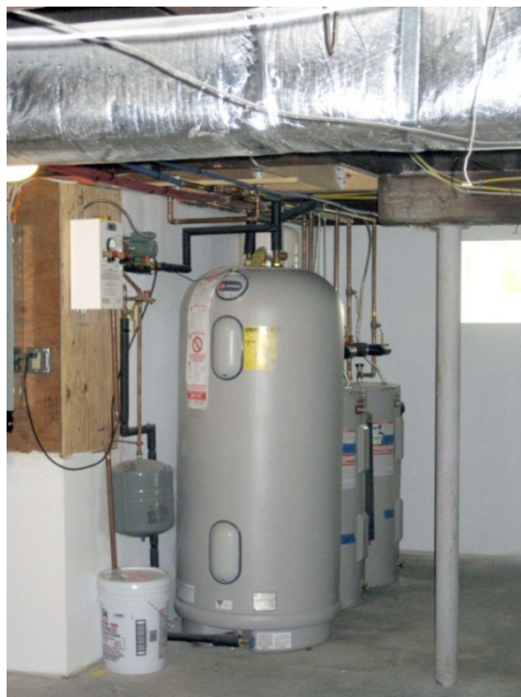
Figure 11. Belmont Two-Family DHW storage tank for solar thermal with backup electric tanks
