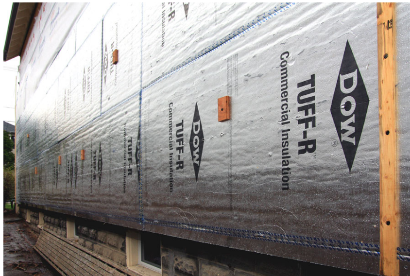
Figure 2. Insulating sheathing on the Belmont Two-Family
