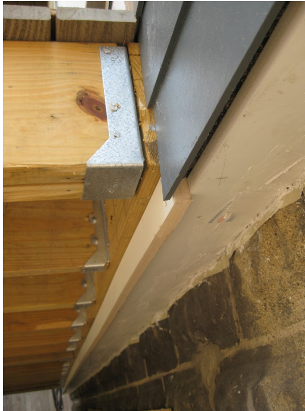
Figure 8. Belmont Two-Family porch deck attachment (from below)
