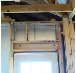
(Top) Rigid foam exterior sheathing is taped to provide an air seal and moisture barrier as well as additional insulation value.
