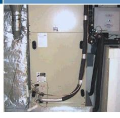
The first-generation zero-energy home contains an AC unit and an integrated solar water and space heating system. In the second-generation home, solar collectors provide water heating with backup water heating provided by a tankless gas water heater and space heat provided by an air source heat pump (Photo source: by NAHBRC).
