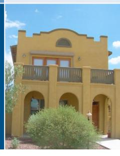
John Wesley Miller combined thick masonry walls with rigid foam sheathing insulation, R-38 attic insulation, high-performance windows, 14-SEER heat pumps, with solar photovoltaic and water heating systems for 50% energy savings over the Building America benchmark on all 97 standard units at Armory Park del Sol in Tucson.
