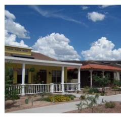
Deep overhangs and porches help minimize heat gain to the interior of the home. Xeriscaping minimizes irrigation needs in the hot dry climate.
