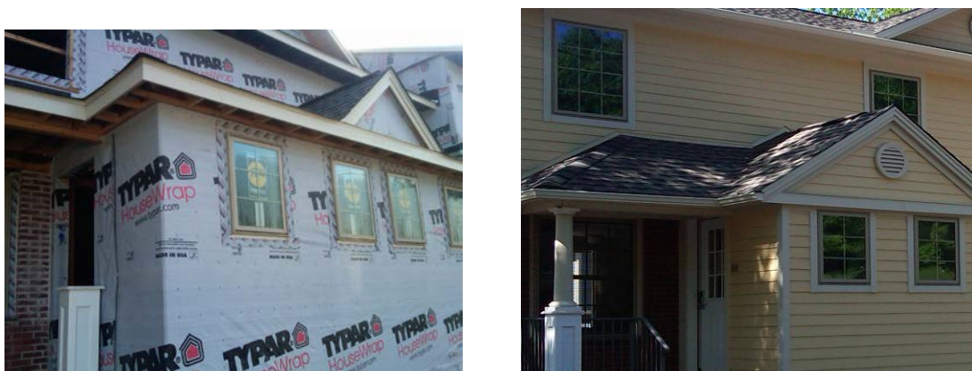
Figure 13. Windows during and after retrofit
