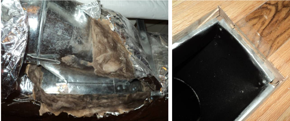
Figure 21. Basement ducts were unsealed in initial units
