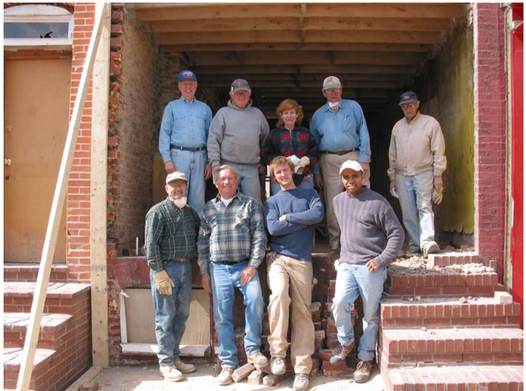
Chesapeake Habitat for Humanity volunteers gather in front of a recently deconstructed row house on West Cross Street.
