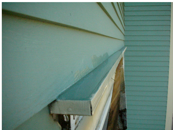
Improper sloped head flashing directing water back towards the building
