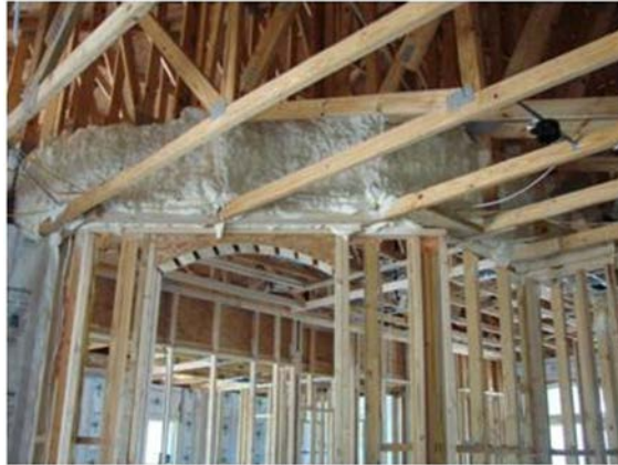
Figure 7. Foam applied to knee wall in attic where ceiling heights transition from 8 to 10 ft
