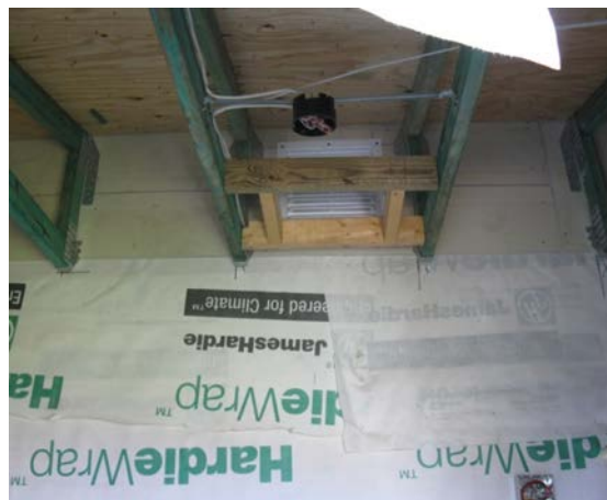
Figure 12. Closet under construction. Grille on back wall connects attic space of closet to vented attic of house through gable end. Rough framing can be seen for grille in closet ceiling that will complete connection between closet and attic.
