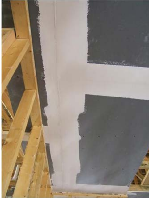
Figure 4. Drywall is also offset beyond the wall/chase to allow for marrying adjacent drywall
