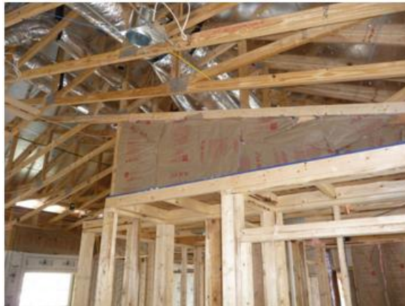
Figure 10. Batt insulation installed to backer board from Figure 9; six-sided sealing of cavity is provided by backer, facing drywall (yet to be installed), and framing members
