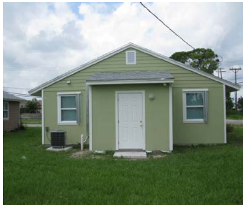
Figure 11. Completed exterior HPWH closet
