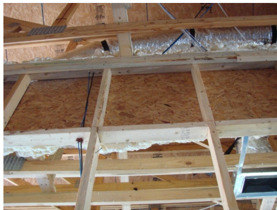
Figure 6. Backside of a foamed knee wall, showing blocker board used to serve as backing for the foam
