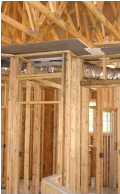
Figure 1. FDC after rough framing
