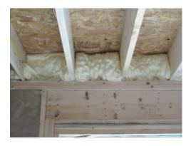
For air barrier purposes, spray foam must connect from first floor wall top plate, up rim joist, and to floor sheathing; of course, connections to remainder of air barrier system (e.g., Air Drywall Approach) must be made.
