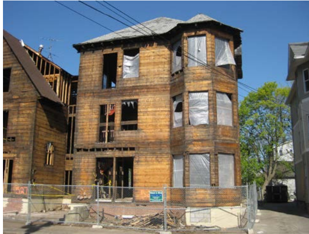
Figure 12. Exterior finishes are removed and existing wall sheathing is exposed.
