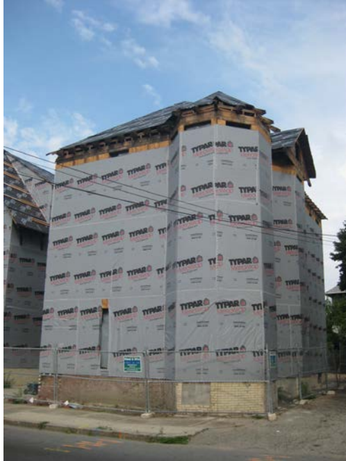
Figure 14. Water- and air-control membrane is in place.
