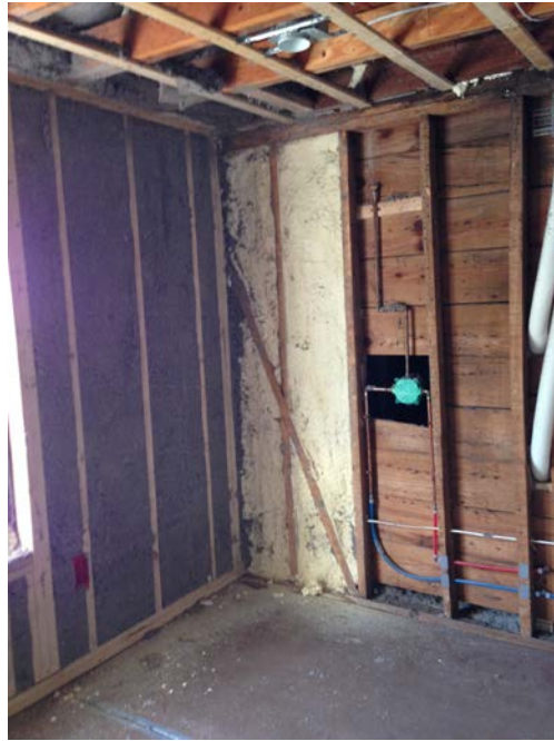
Figure 18. ccSPF and cellulose insulation
