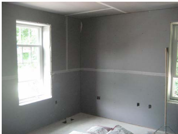
Figure 19. New gypsum board installed
