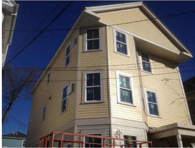
Figure 16. Completed cladding and trim
