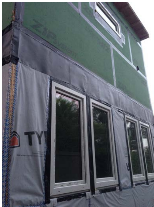
Figure 15. Windows are installed after openings are flashed.
