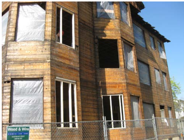
Figure 13. Windows and doors are removed.
