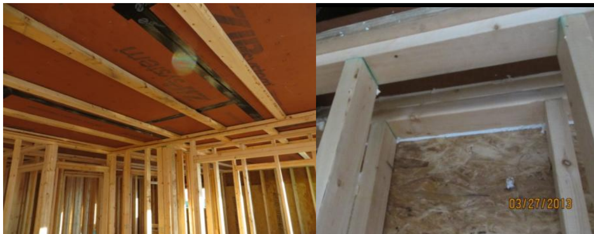
Figure 7. The ceiling air barrier was created with sheathing (left) and then furred out to provide a chase for wiring to prevent penetrations into the attic. Crews aggressively sealed the top plate with caulk (right).
