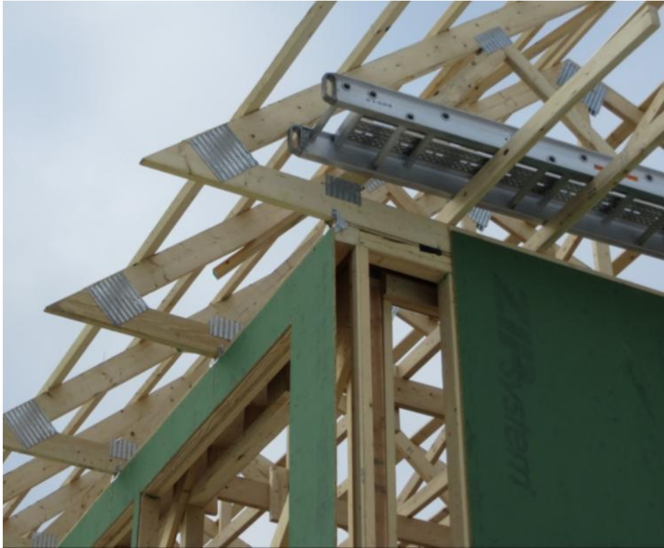
Figure 6. Exterior top plate connections are hard to properly seal due to interruption of roof ties
