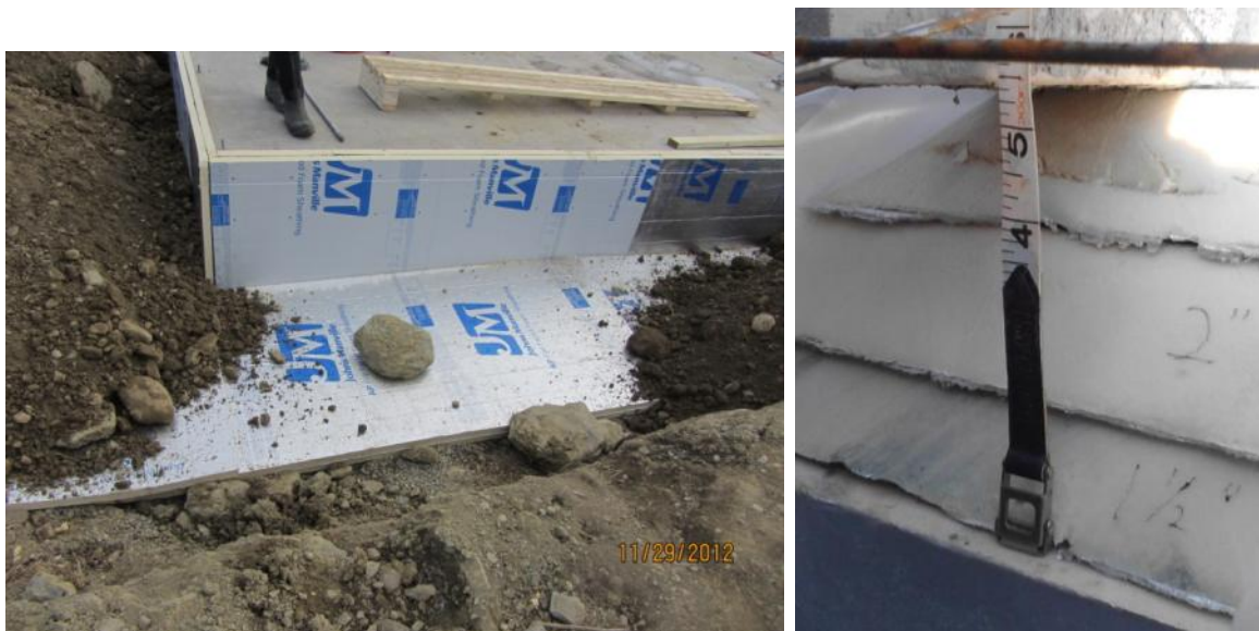
Figure 3. Slab edge (left) and under slab insulation (right) at TREE
