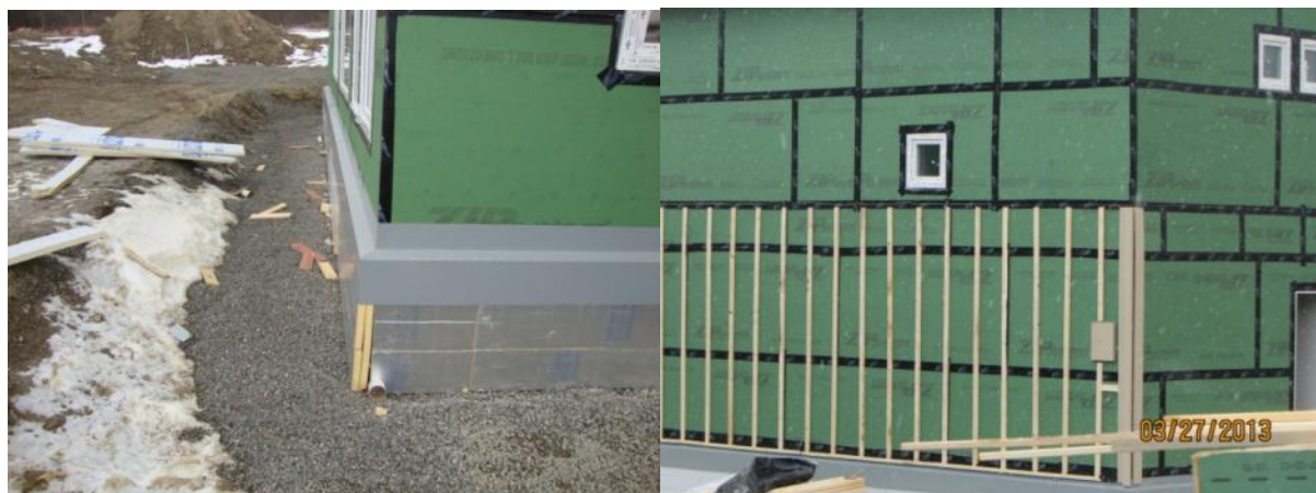
Figure 8. Flashing over slab edge insulation was taped to sheathing using the manufacturer's approved tape. The vented cladding was then attached with \frac{3}{4} in. furring strips and overlapped the flashing.
