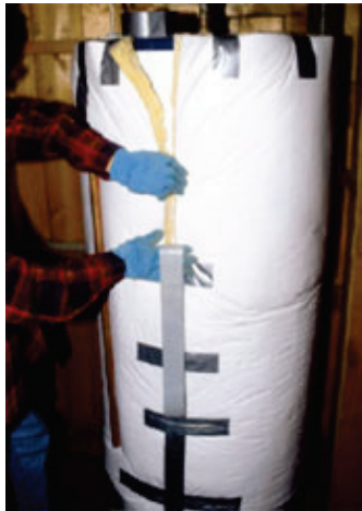
Figure 19. Water heater insulating blanket
