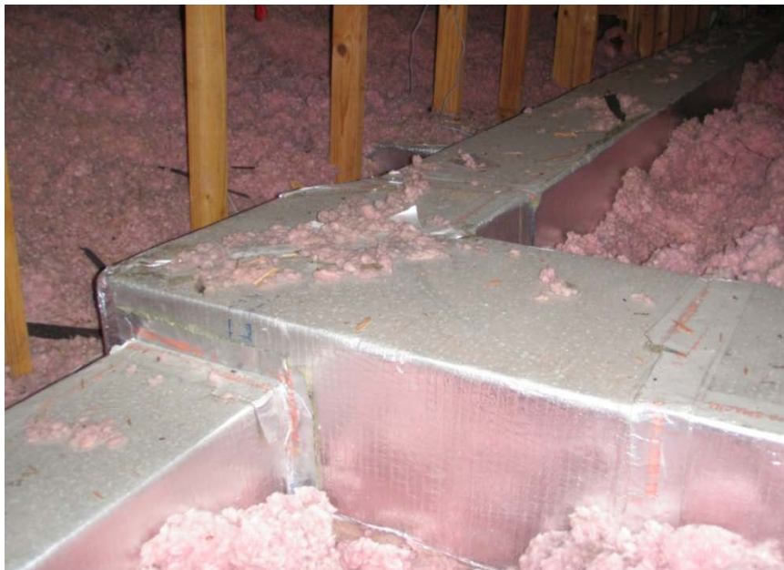
Figure 8. Supply ductwork for House 2
