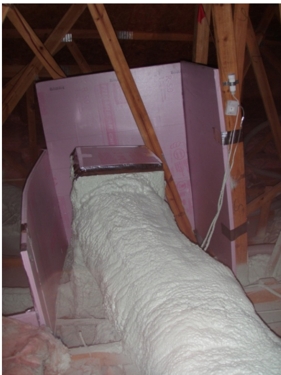
Figure 14. Baffling used to ensure proper burial of supply duct plenum (post-encapsulation and pre-burial)
