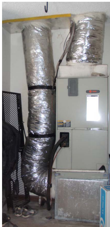
Figure 24. AHU at House 2 located in garage with leaky return and supply plenums
