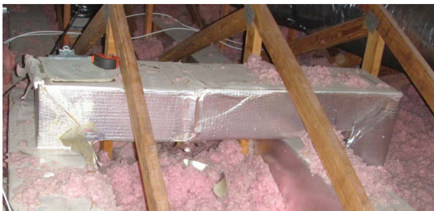
Figure 10. Supply ductwork jump over abandoned return ductwork
