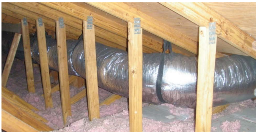
Figure 9. Return ductwork for House 2
