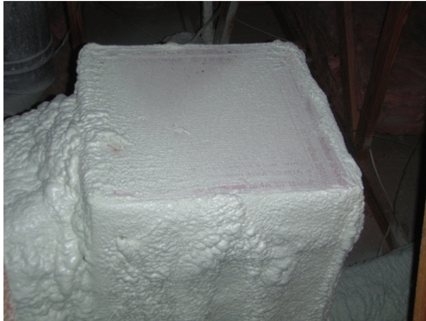
Figure 17. Improperly spray-foamed plenum box at House 1
