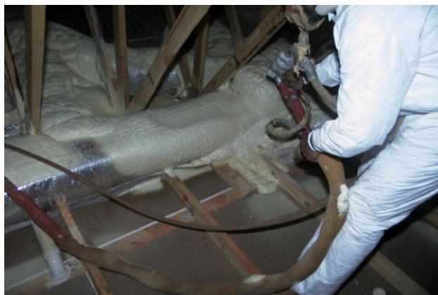
Figure 2. Ducts being encapsulated with ccSPF
