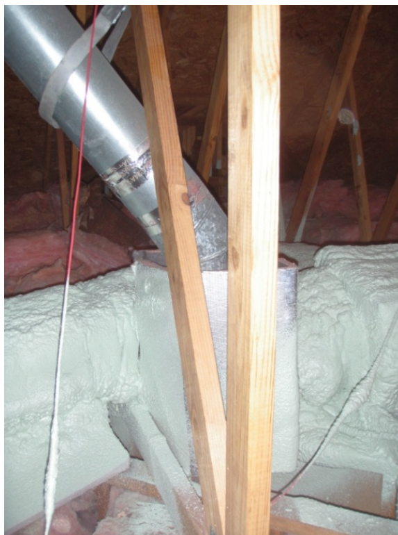
Figure 15. Baffling used to prevent ccSPF application on flue duct
