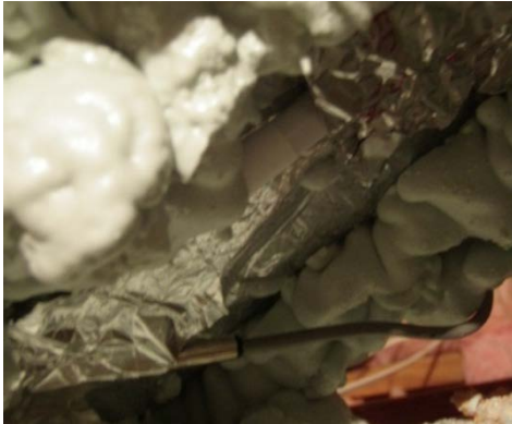
Figure 18. Exposed duct jacket at the underside of duct
