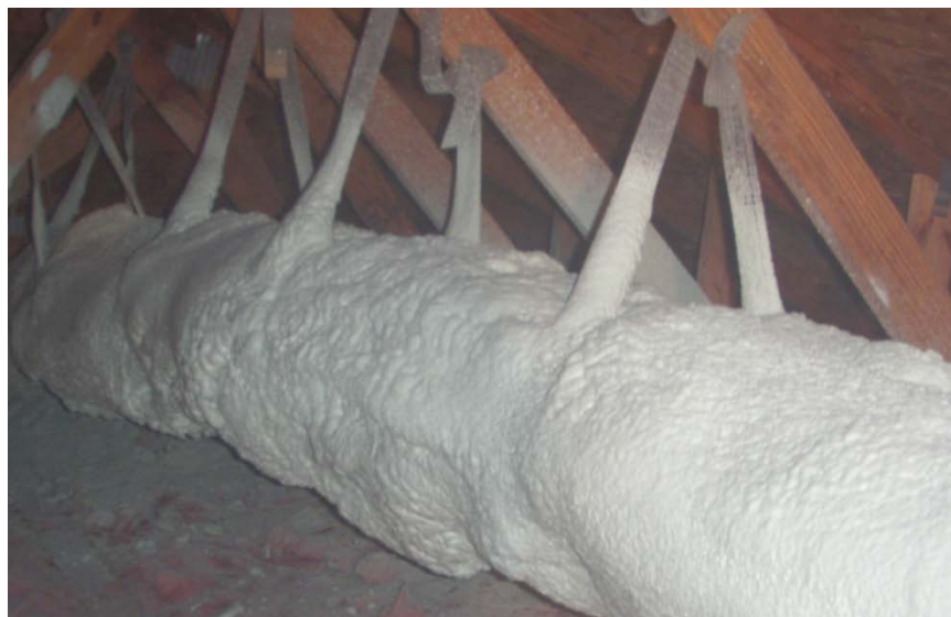
Figure 13. Finished encapsulated duct hung from roof deck
