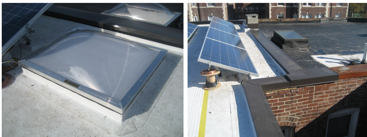
Figure 22. Skylight installation (left) and metal cap flashing (right)
