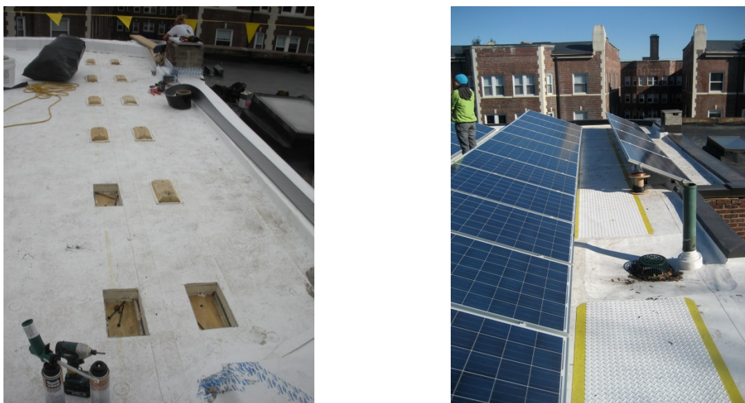
Figure 20. Roof membrane with blocking for PV system rack (left); finished roof (right)
