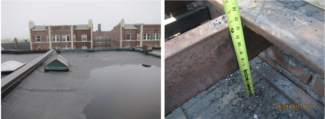
Figure 13. Existing roof cladding to be removed (left) and verification of existing conditions (right)
