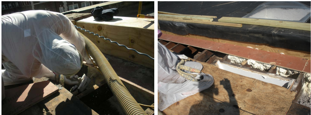
Figure 15. Spray foam installation connecting masonry wall to roof sheathing (air barrier)
