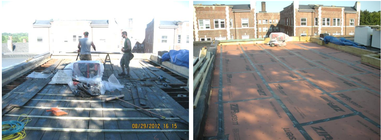
Figure 17. Sleepers over existing board sheathing (left); new roof sheathing at field of roof (right)
