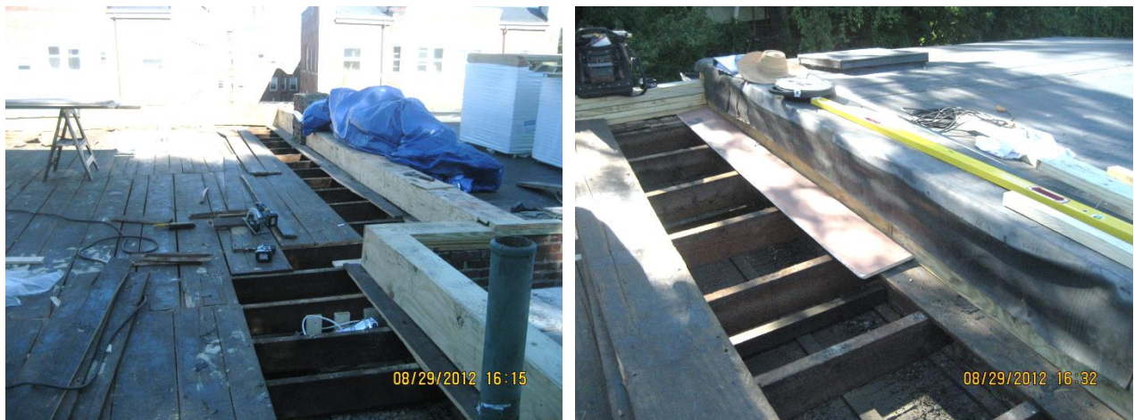
Figure 14. Existing boards removed near roof perimeter with pressure-treated plywood installed at parapet (left); strip of OSB sheathing with integrated water-resistant barrier at parapet (right)
