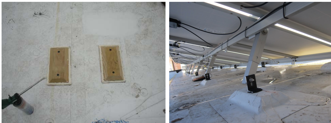
Figure 21. PV system rack attachment during construction (left) and installation completed (right)
