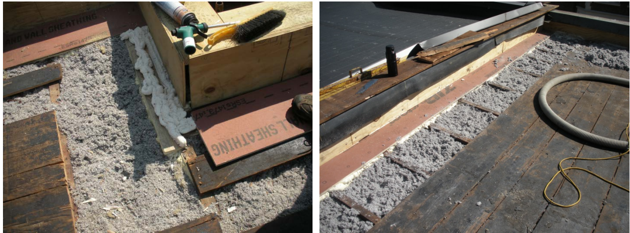
Figure 16. Fibrous insulation installed in the rafter cavity with air sealing details
