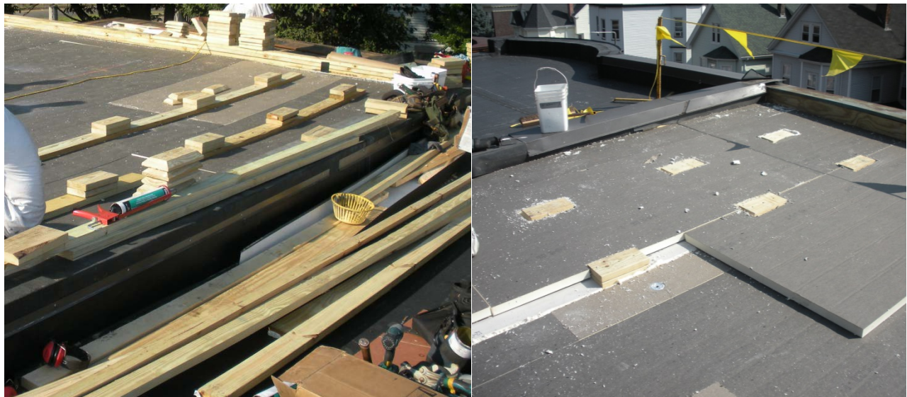
Figure 19. Blocking for future PV installation
