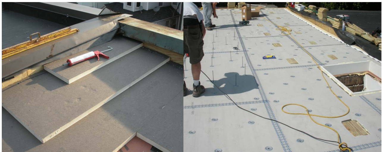
Figure 18. Rigid insulation in multiple layers with staggered seams (left); insulation cover board (right)
