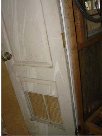
Figure 26. Interior closets that served as return plenums had louvered doors or door-mounted return grilles.
