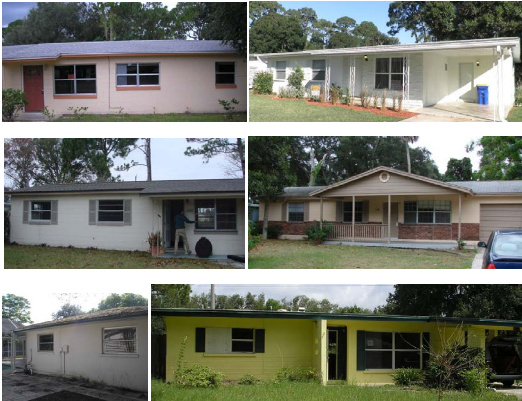
Figure 5. Study homes of typical character with ranch style floor plans, slab-on-grade foundations, concrete block exterior walls, low sloped roofs, and 8-ft ceiling heights
