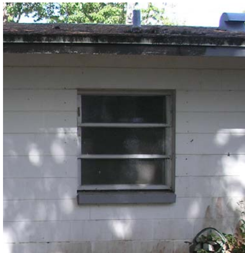
Figure 9. Typical awning-style window type
