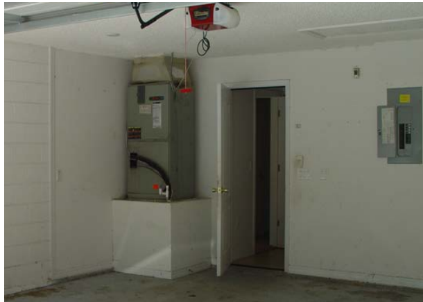
Figure 27. Upflow AHUs on framed platforms in garage with a wall-mounted filter-back grille were ducted directly into the platform cavity.
