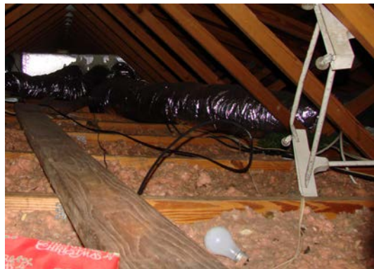
Figure 13. Typical pre-retrofit ceiling insulation condition
