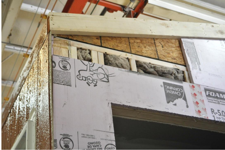
Figure 19. Installing CI at the gable
