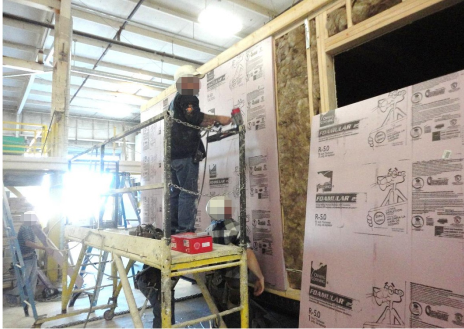
Figure 18. Installing and tacking foam boards
