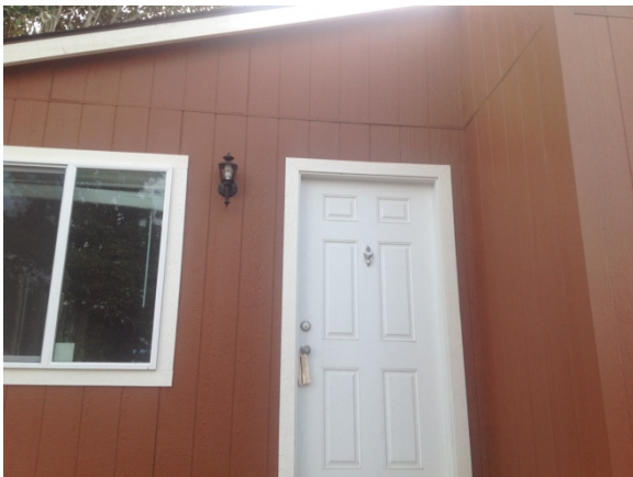
Figure 14. No damage to the exterior walls of the test home: end wall
