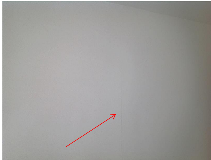
Figure 13. Interior wall crack on the test home
