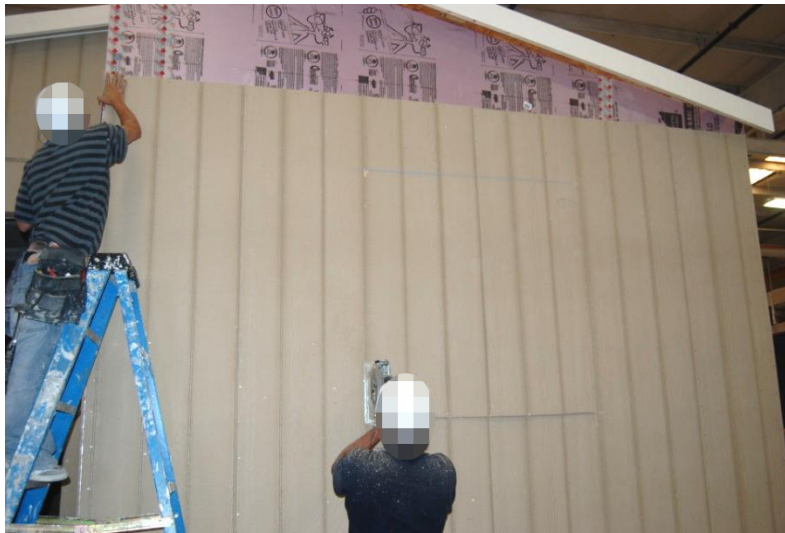
Figure 21. Cutting out a window opening with a circular saw
