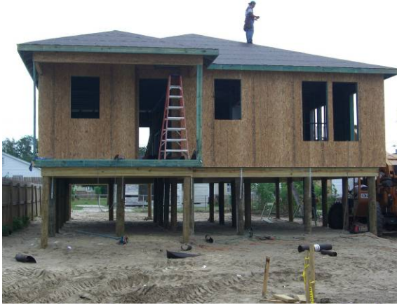
Figure 6. Windstorm OSB installed over the entire wall system as the exterior sheathing
