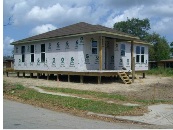
Figure 7. Woven house wrap installed over the exterior sheathing
