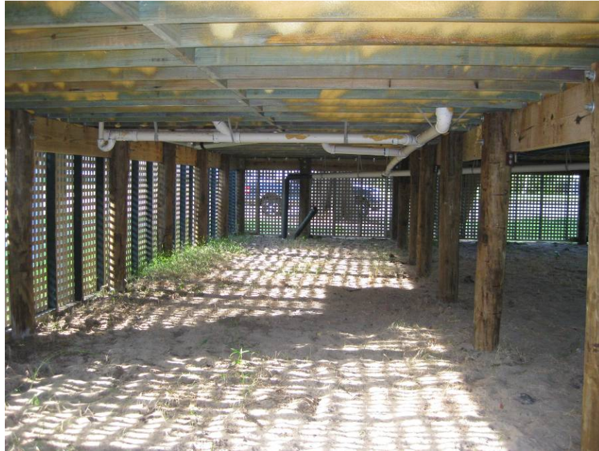
Figure 5. Wood pile foundation system
