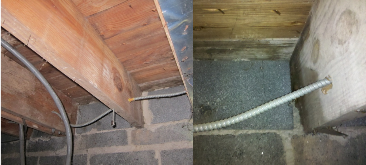
Figure 16. Water-sensitive wood joists embedded into water-absorptive concrete block
