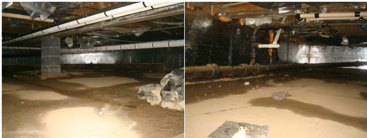
Figure 20. Crawlspace photo showing wetness at seams in the concrete slab (L) and (R), and floor drain backup (L)
