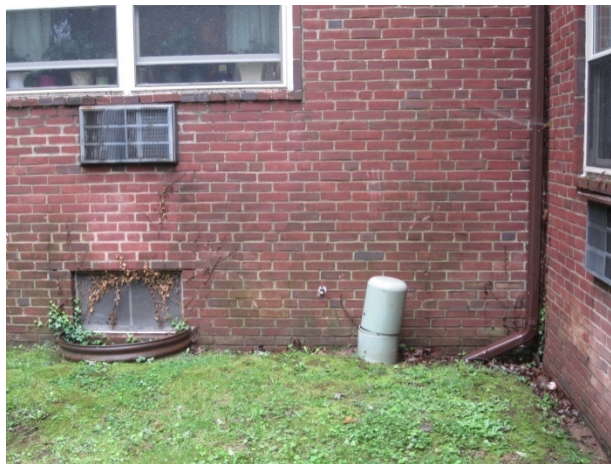
Figure 24. Roof gutter downspout not piped to storm drain system allowing water intrusion to crawlspace
