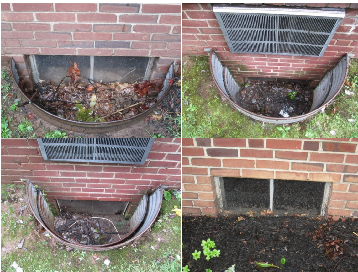
Figure 11. Evidence indicating bulk water intrusion through the crawlspace windows
