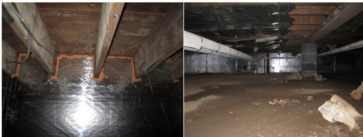
Figure 31. Crawlspace foundation wall insulation fit well and sealed at edges and penetrations (L); some crawlspace conditions remained wet but drying, with exhaust ventilation throughout and sump pumps in critical locations (R)
