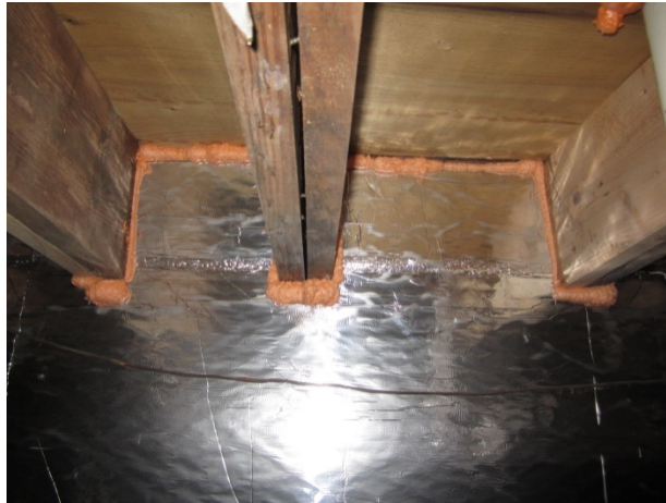
Figure 19. Example of air leakage to unit above but well-sealed foundation wall
