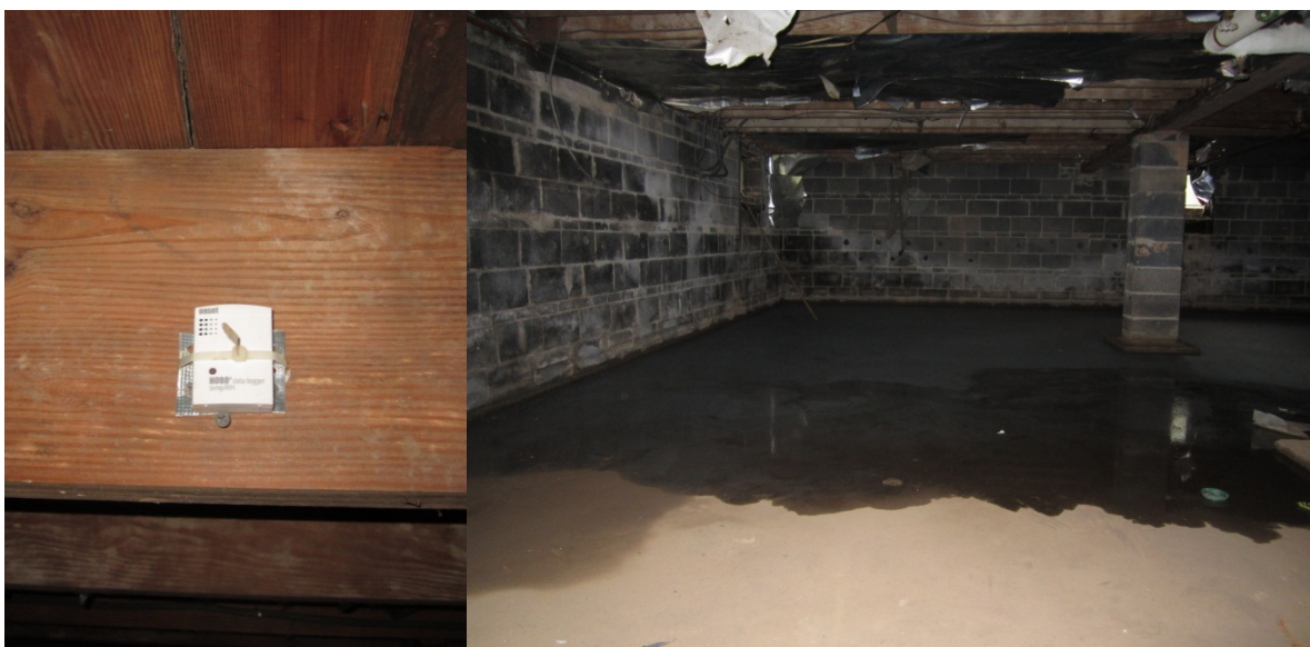
Figure 22. Temperature and RH data logger (L); standing water in crawlspace (R)
