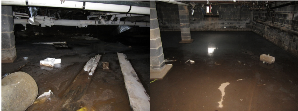
Figure 23. Inaccessible Building B crawlspace (L), and Building E crawlspace (R) with standing water during a rainy period
