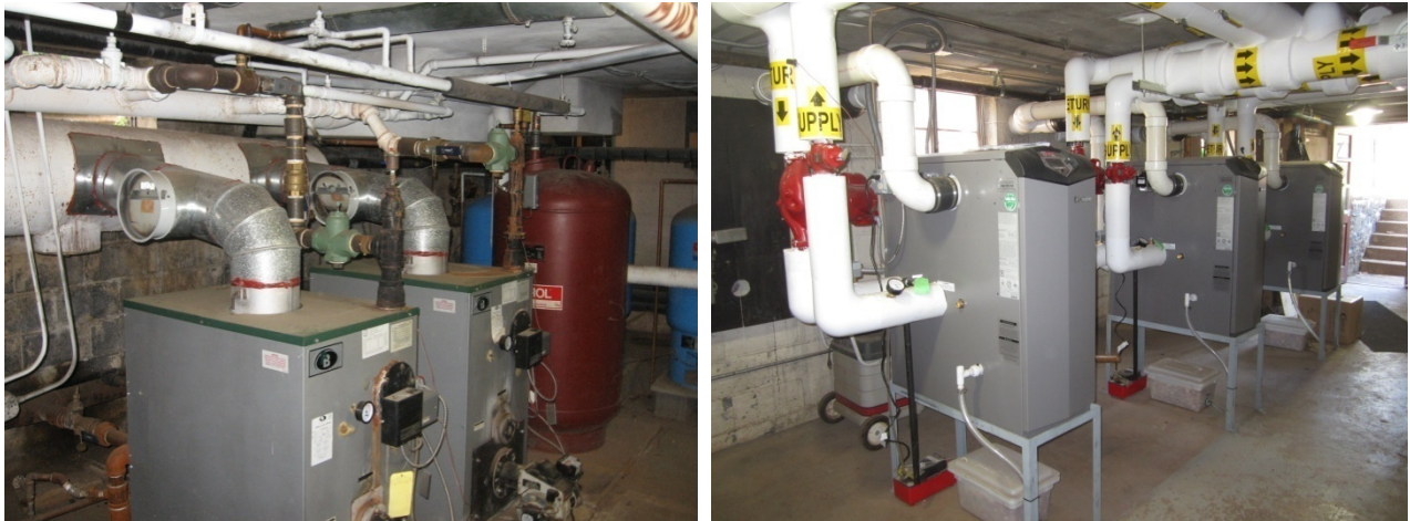
Figure 9. Atmospheric boilers (L) were replaced with condensing sealed-combustion boilers (R)
