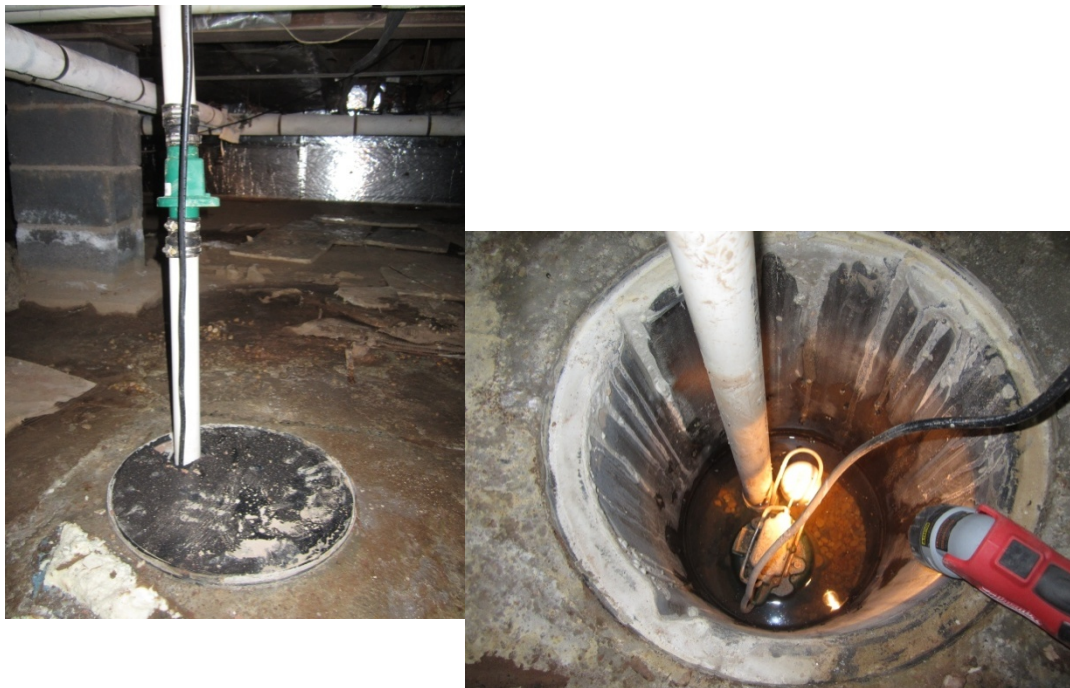
Figure 34. Sump pump installation; sides of sump pit are perforated with drilled holes, but perforating the bottom would be better; concrete debris and mud left in sump should be cleaned out to allow pump impeller to work freely.
