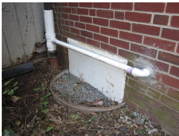
Figure 35. Sump pump water discharged into the roof drain water system
