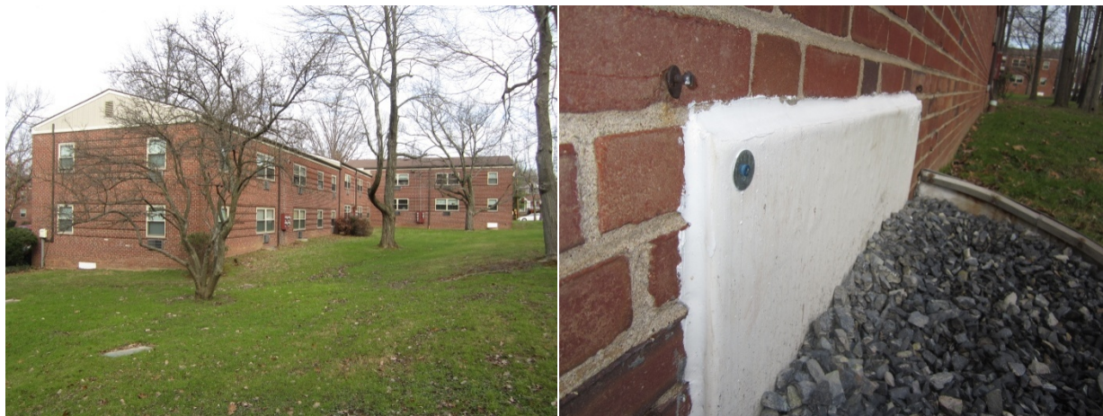
Figure 30. Crawlspace window well blocking and sealing on the back sides of Buildings A and B (L); note the sloped sealant to shed water at the top of the blocking panel (R)
