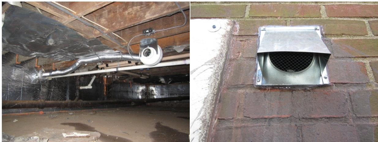
Figure 33. Unvented crawlspace exhaust ventilation fan and ducting to outside wall cap
