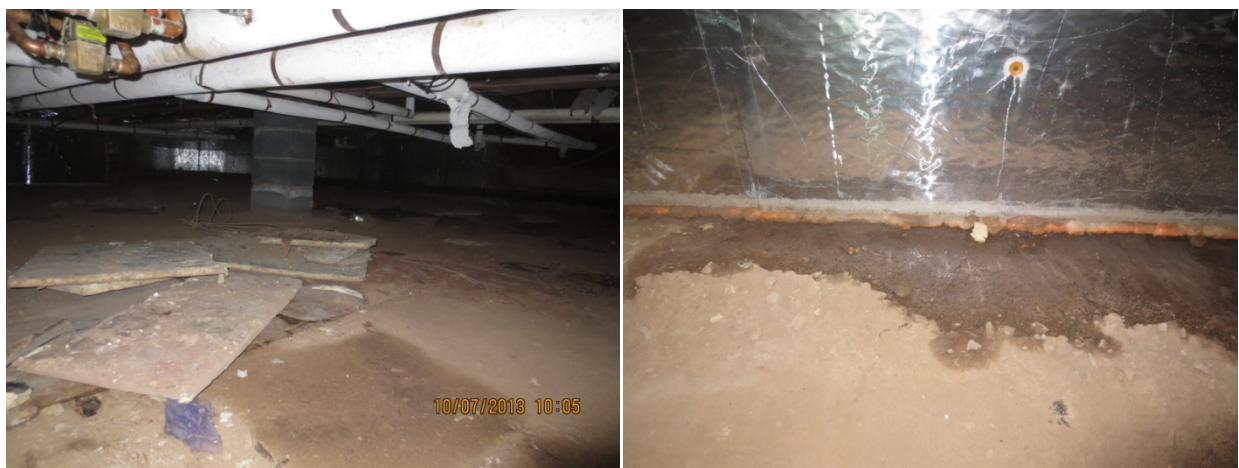
Figure 37. Example of debris and mud, holding moisture in crawlspace (L); example of small area of standing water at slab edge and foundation wall (R)
