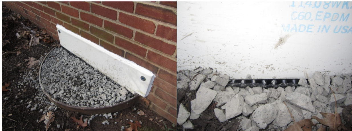
Figure 29. Finished view of the crawlspace window blocking retrofit to eliminate that bulk water intrusion (L); note the foundation drainage mat protecting the waterproof membrane (R)
