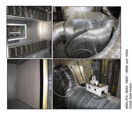
Figure 2. Duct heaters used to control humidity (top left), heat exchanger to provide cooling (top right), evaporation pads (bottom left), and temperature and humidity measurement at inlet to plenum (bottom right)
