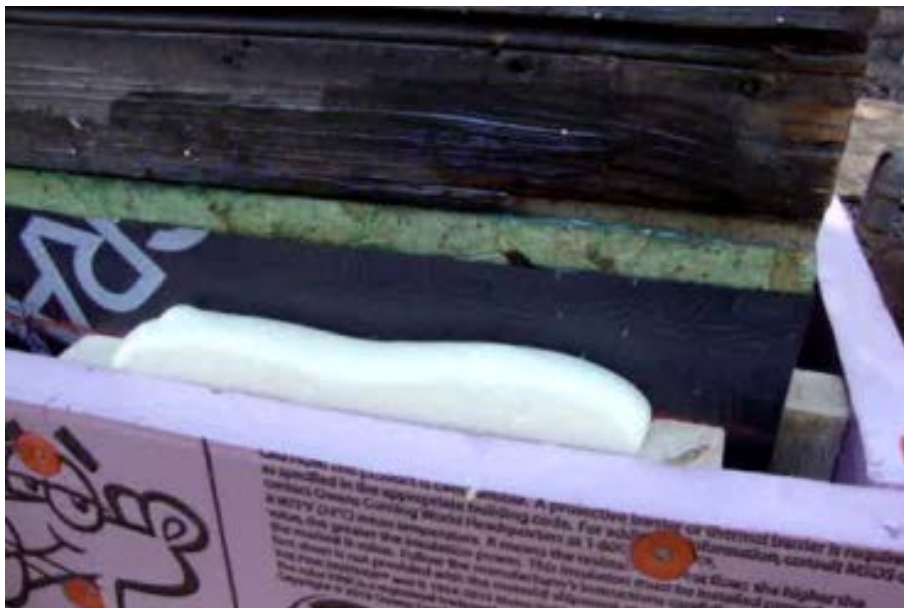
Figure 20. View of above-grade wall after liquid foam was added
