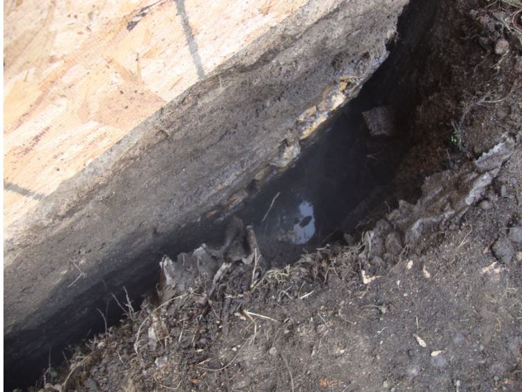
Figure 12. Debris encountered during trenching
