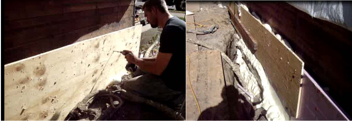
Figure 21. Temporary plywood to control foam expansion
