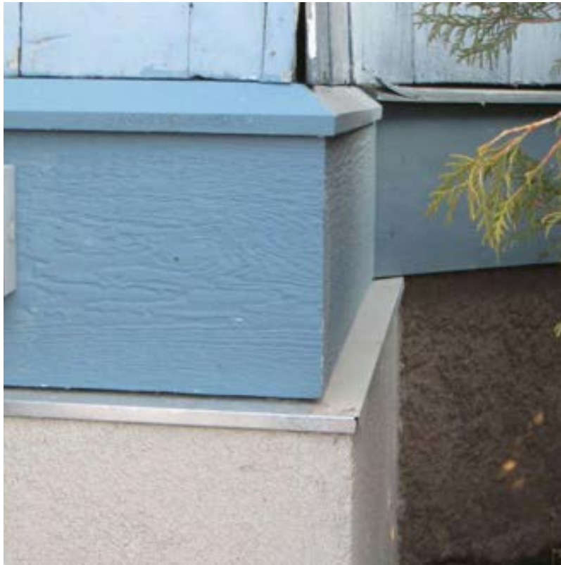
Figure 23. Step design at wall/rim transition
