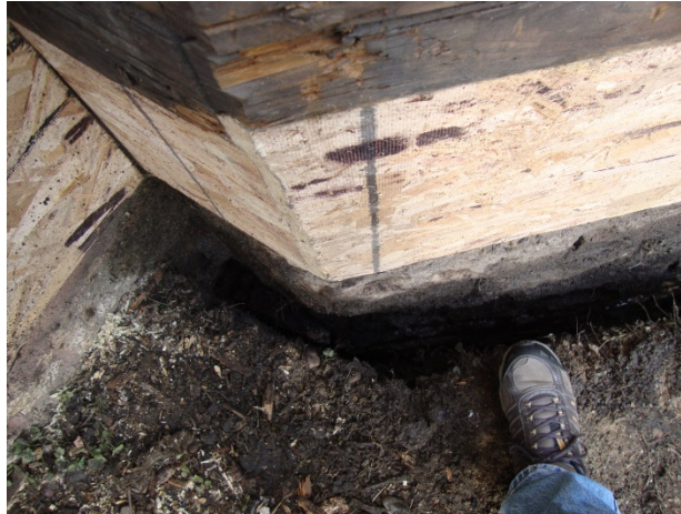
Figure 10. The trench after vacuuming
