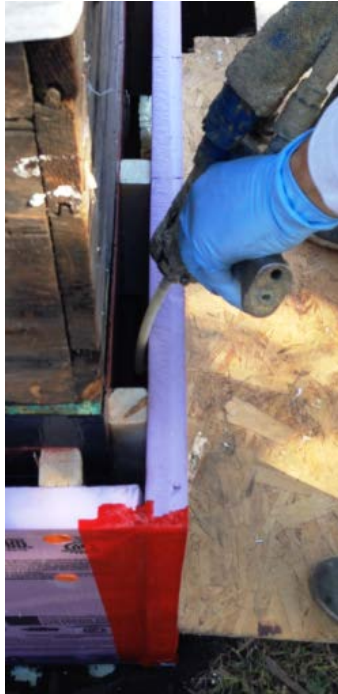
Figure 19. Liquid foam dispensed between wall and XPS
