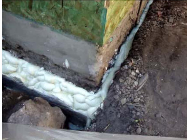
Figure 15. Foam terminated 6–12 in. BG
