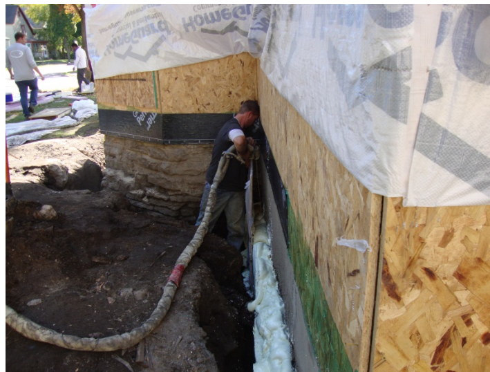
Figure 16. Rigid panel used to contain liquid foam in areas of soil collapse
