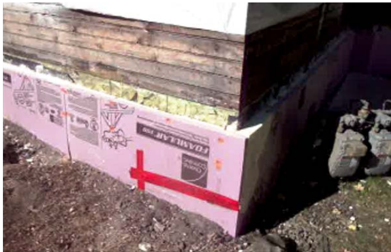
Figure 22. Final result of XPS/liquid foam AG insulation
