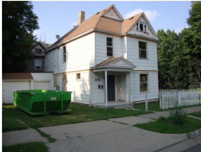
Figure 4. Subject house in north Minneapolis prior to renovation
