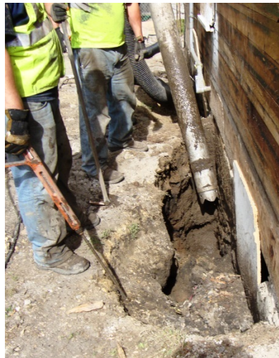
Figure 11. Soil collapse being cleared by vacuum
