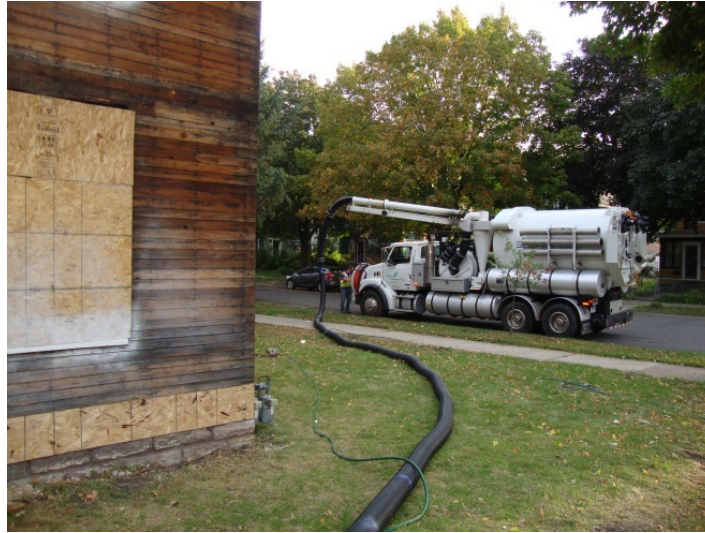
Figure 6. The vacuum hose and truck-mounted pressurized water system
