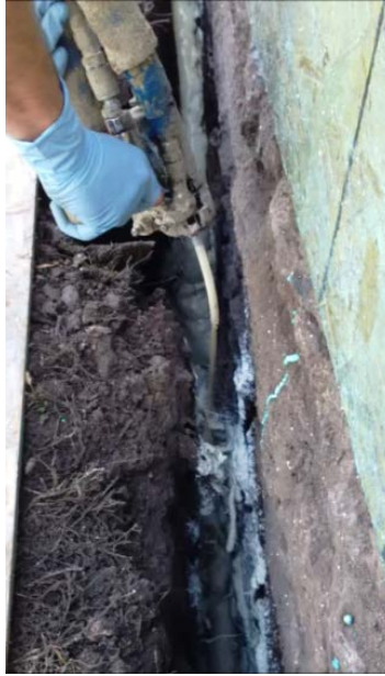
Figure 13. Dispensing liquid foam
