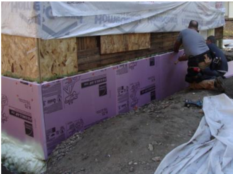
Figure 18. Smooth XPS foam board attached to wood standoffs
