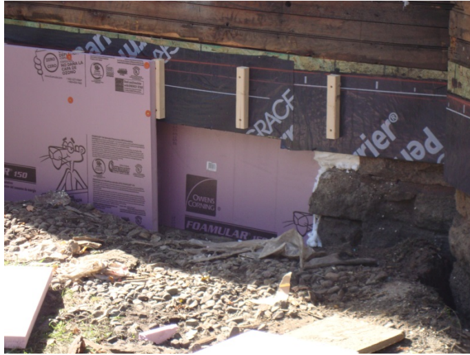
Figure 17. Wood standoffs attached to rim
