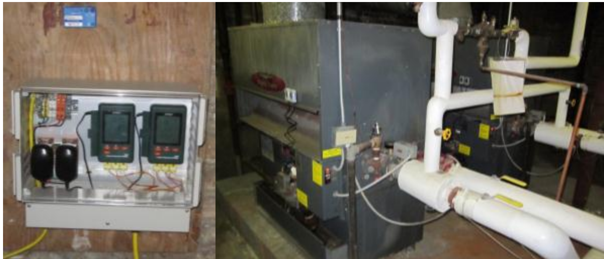
Figure 8. Chicago site—TC logger in room A (right) and monitored boilers in room B (left)
