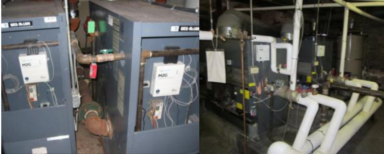
Figure 7. M2G-equipped boilers at Cary (left) and Chicago (right) sites
