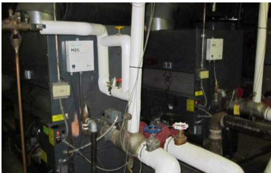
Figure 1. M2G-equipped boilers at test site
