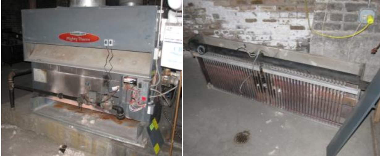
Figure 9. Damaged boiler #1 at Chicago site A with removed burner assembly (right)
