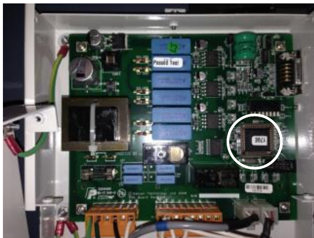
Figure 12. M2G control board with replaced chip at Cary site (circled)
