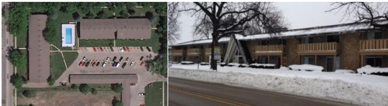
Figure 6. Aerial view and photograph of Cary site
