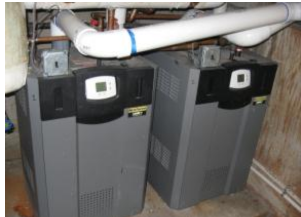
Figure 4. Incompatible boilers at Cicero site
