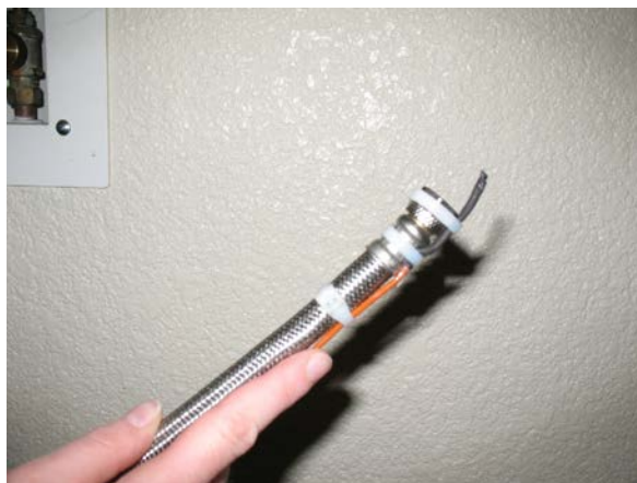
Figure 38. Thermocouple to measure end-use temperature of hot water
