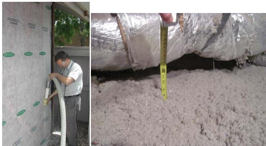
(a) Dense pack blown-in cellulose being installed in the west wall. Credit: Judy Lew-Loose, SMUD.
