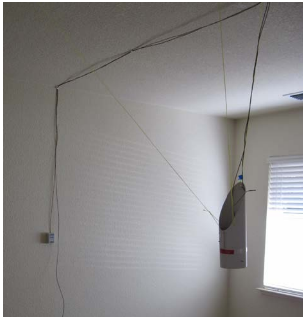
Figure 58. Thermocouples for interior temperature measurements
