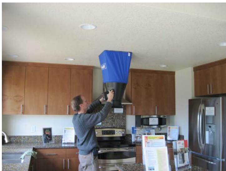
Figure 9. Flow hood test in progress
