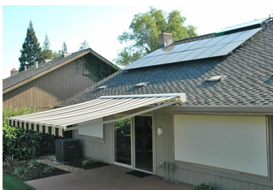
(a) The motorized exterior shading and awning on the west side of the house. Credit: Judy Lew-Loose, SMUD
