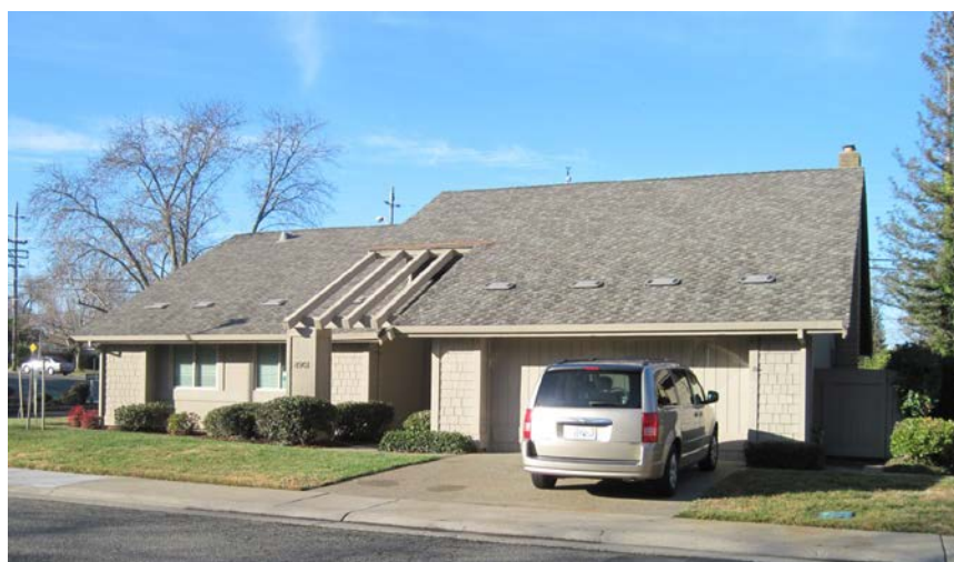
Figure 1. The Greenbuilt house
