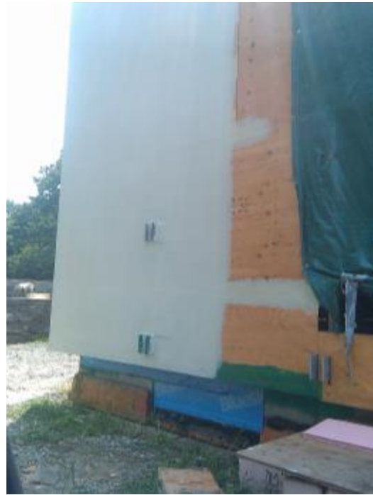
Figure 19. Image of liquid-applied WRB
