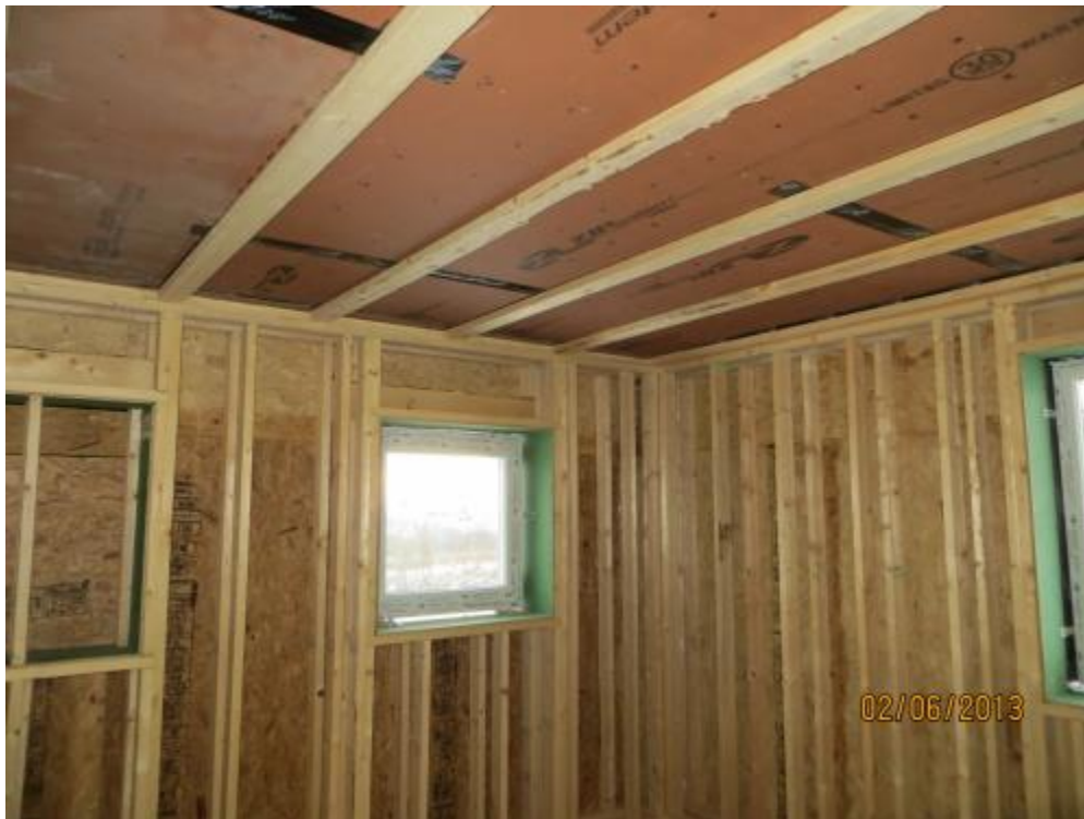
Figure 1. Double-wall construction
