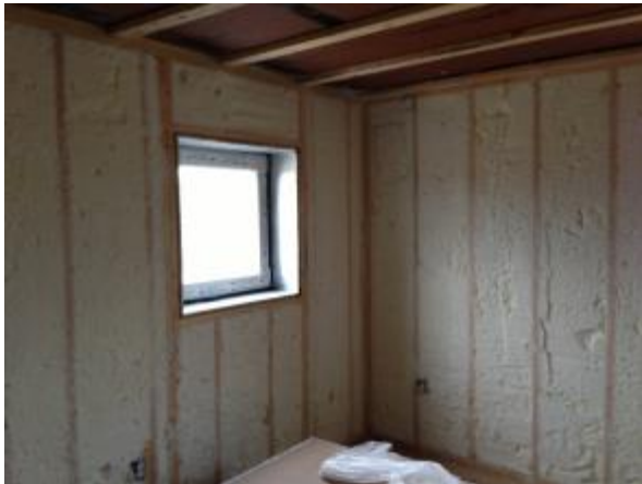
Figure 2. ocSPF in a 12-in. double wall
