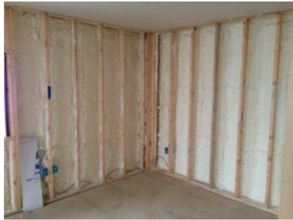
Figure 3. ccSPF in the outer stud cavity of a 12-in. double wall. Cellulose will fill the remainder of the cavity.
