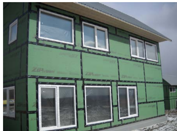
Figure 15. Exterior air barrier with all seams taped
