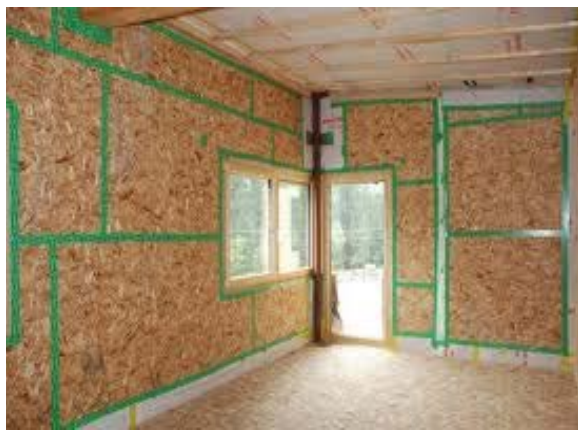
Figure 14. Interior air barrier with all seams taped
