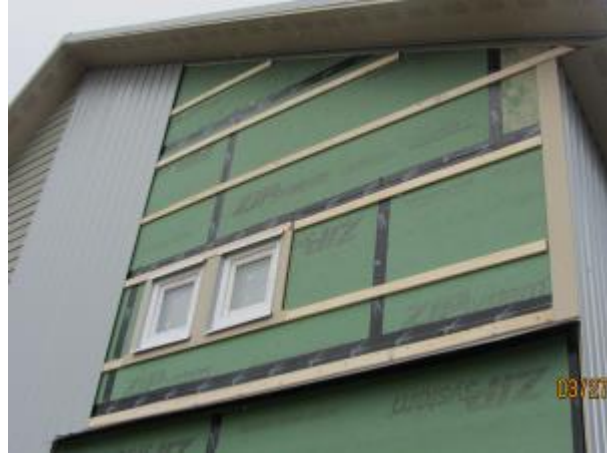
Figure 21. Horizontal furring was used to attach a corrugated metal panel siding that allows vertical draining and venting of the sheathing.
