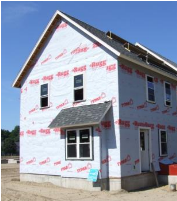
Figure 18. Example of a building wrap being used for the WRB
