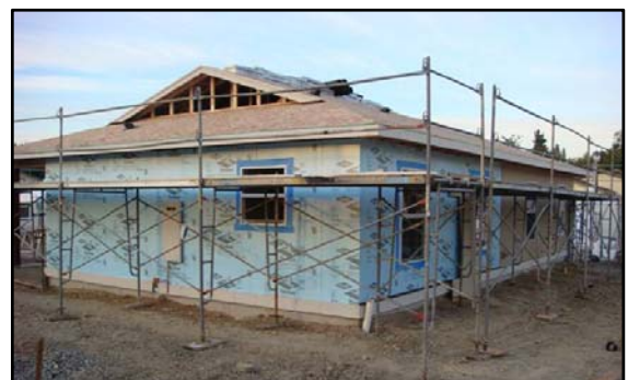
3. ONE INCH EXPANDED POLYSTYRENE FOAM APPLIED TO OSB SHEATHING TO PROVIDE CONTINUOUS THERMAL BREAK AND ADDITIONAL R-5 WALL INSULATION
