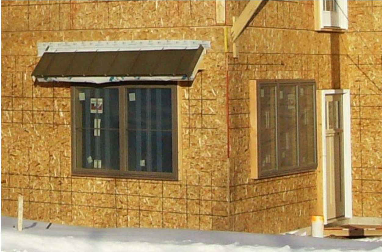
Figure 7. Outset window installation.
