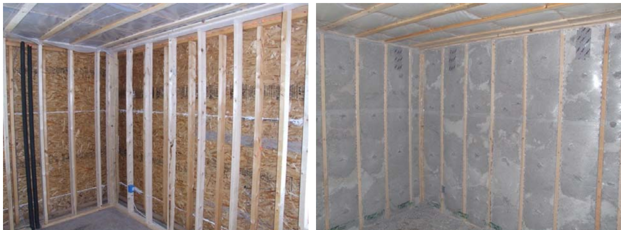
Figure 3. Double wall before and after insulation with dense, blown cellulose.
