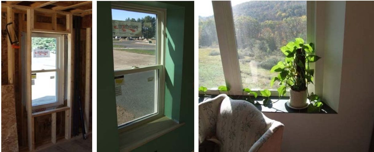
Figure 2. Windows in double walls. From the left: a framed window opening with square returns; a finished window with square returns; a finished window with 45° returns.
