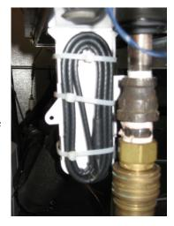
Figure 5. Heat tape on a condensate trap
