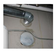
Figure 13. Seal unused vent openings
