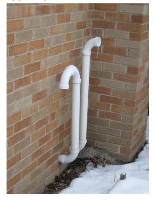
Figure 12. Vent termination above the snow line
