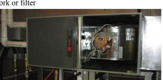
Figure 9. Attic installations are typically horizontal left or right
