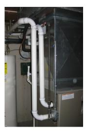
Figure 10. All services may be connected on the same side of the furnace
