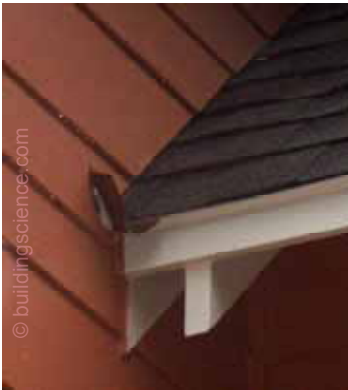
Figure 3. Kick-out flashing at roof-wall intersection
