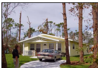
After Hurricane Charley
