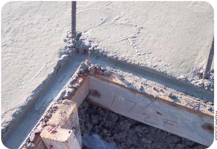
The recessed seat at the edge of the floor slab makes it more difficult for storm-driven water to penetrate the joint between the concrete walls and the floor slab.
