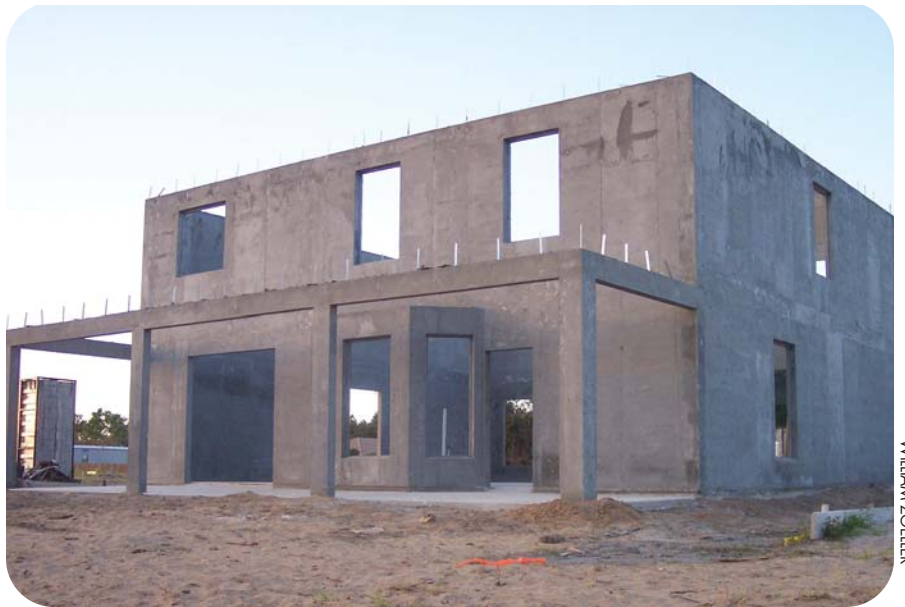
SWA and Mercedes continue to collaborate on hurricane-resistant homes, including this two-story concrete prototype currently under construction.
